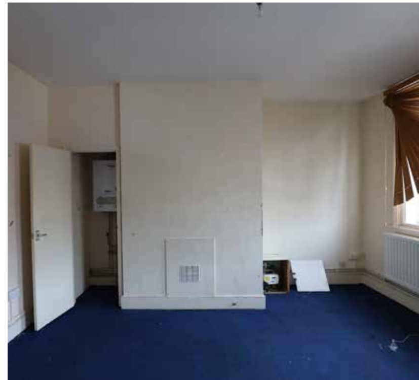
FIGURE 29. First Floor SW Room
