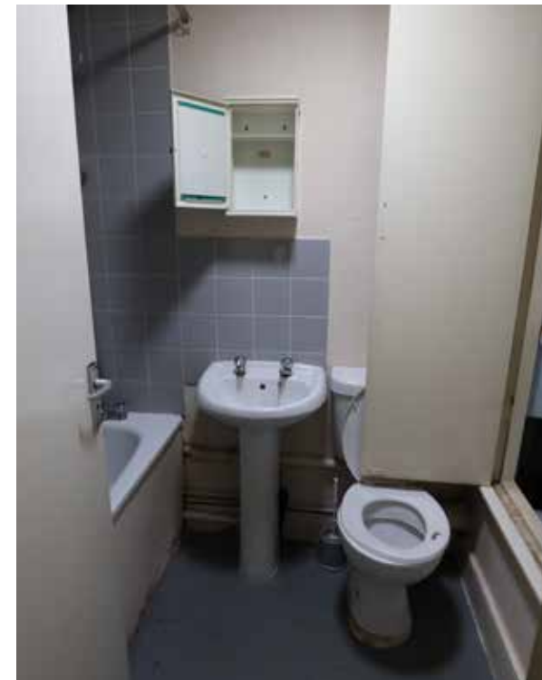
FIGURE 30. Second Floor NE WC
