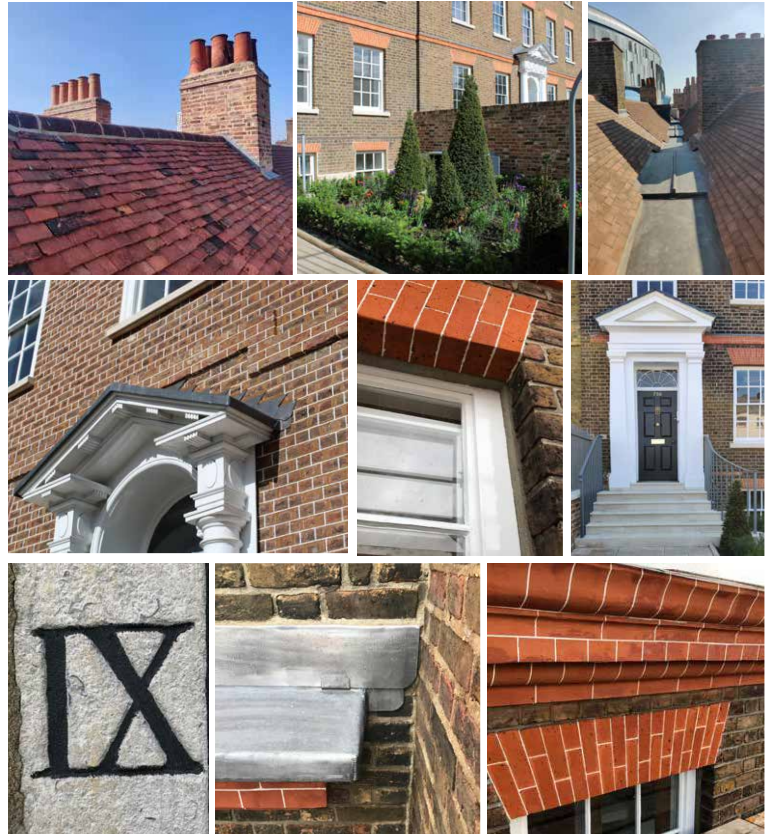
FIGURE 8. External Restoration Works to Northumberland Terrace - Complete March 2022
