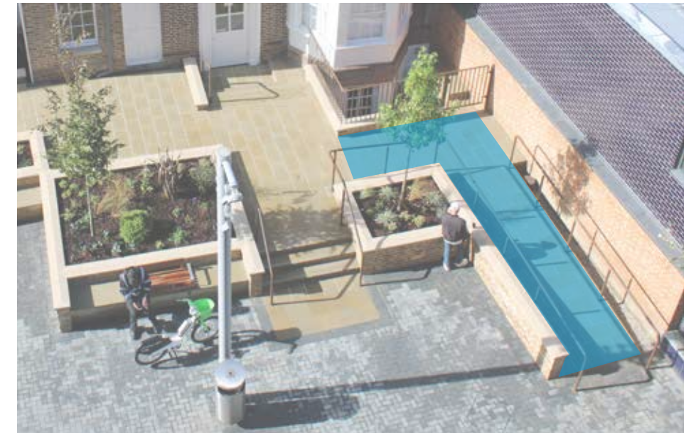
FIGURE 64. Rear View of No. 794
