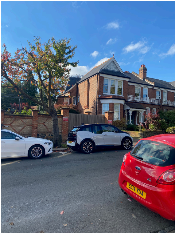
Existing Front elevation photos
