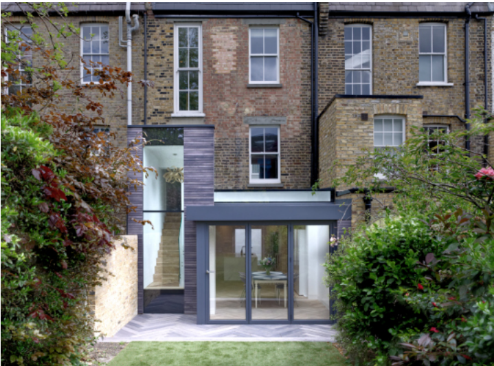
Fig 2. Rear view of Brokesley Street, E3 - Conservation Area, Tower Hamlets
