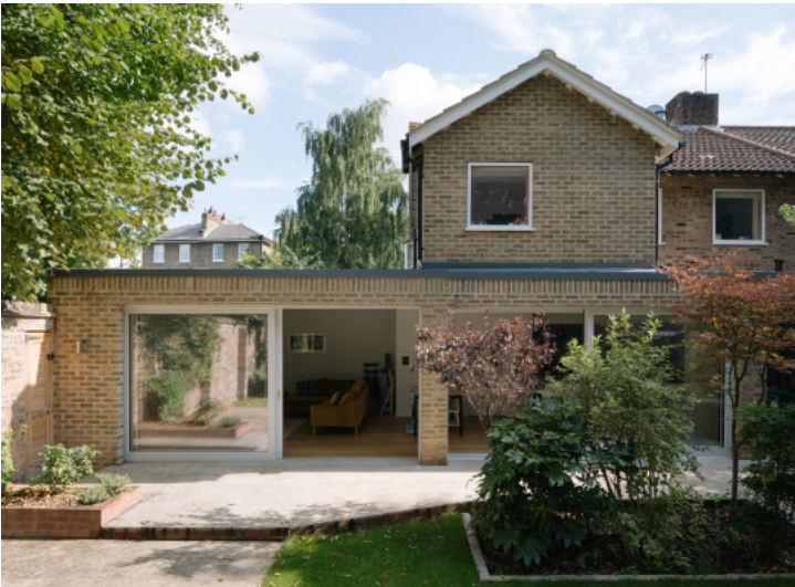
Fig 4. Rear view of Canonbury Park North, N1 - Conservation Area, Islington
