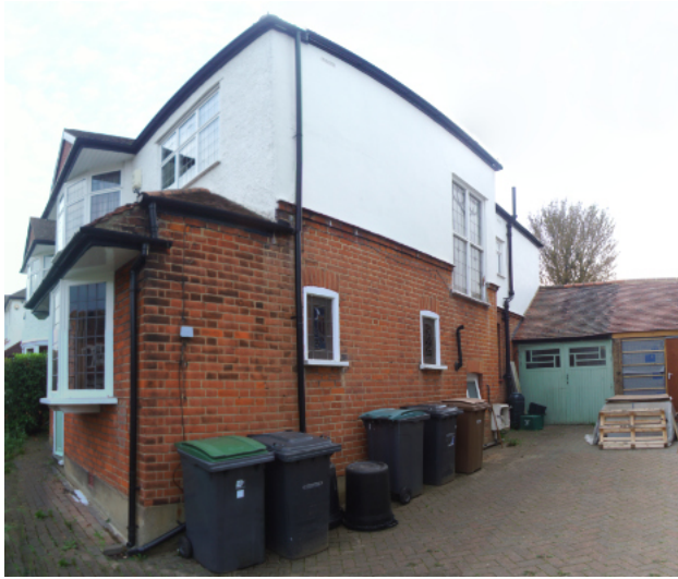
Fig 8. Side view of number 57 &amp; garage
