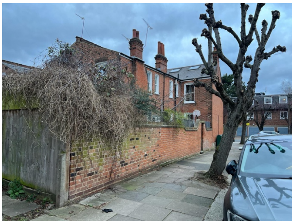
view of side elevation looking towards the corner of Albert Road and Harcourt Road
