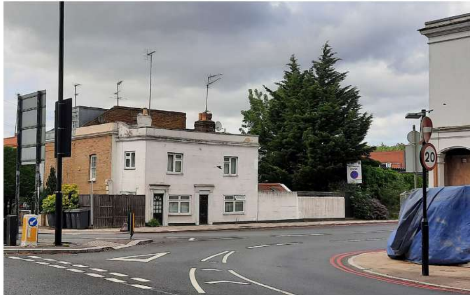
1 Terrace of houses adjacent to the site from the junction of Bakers Lane and North Hill
