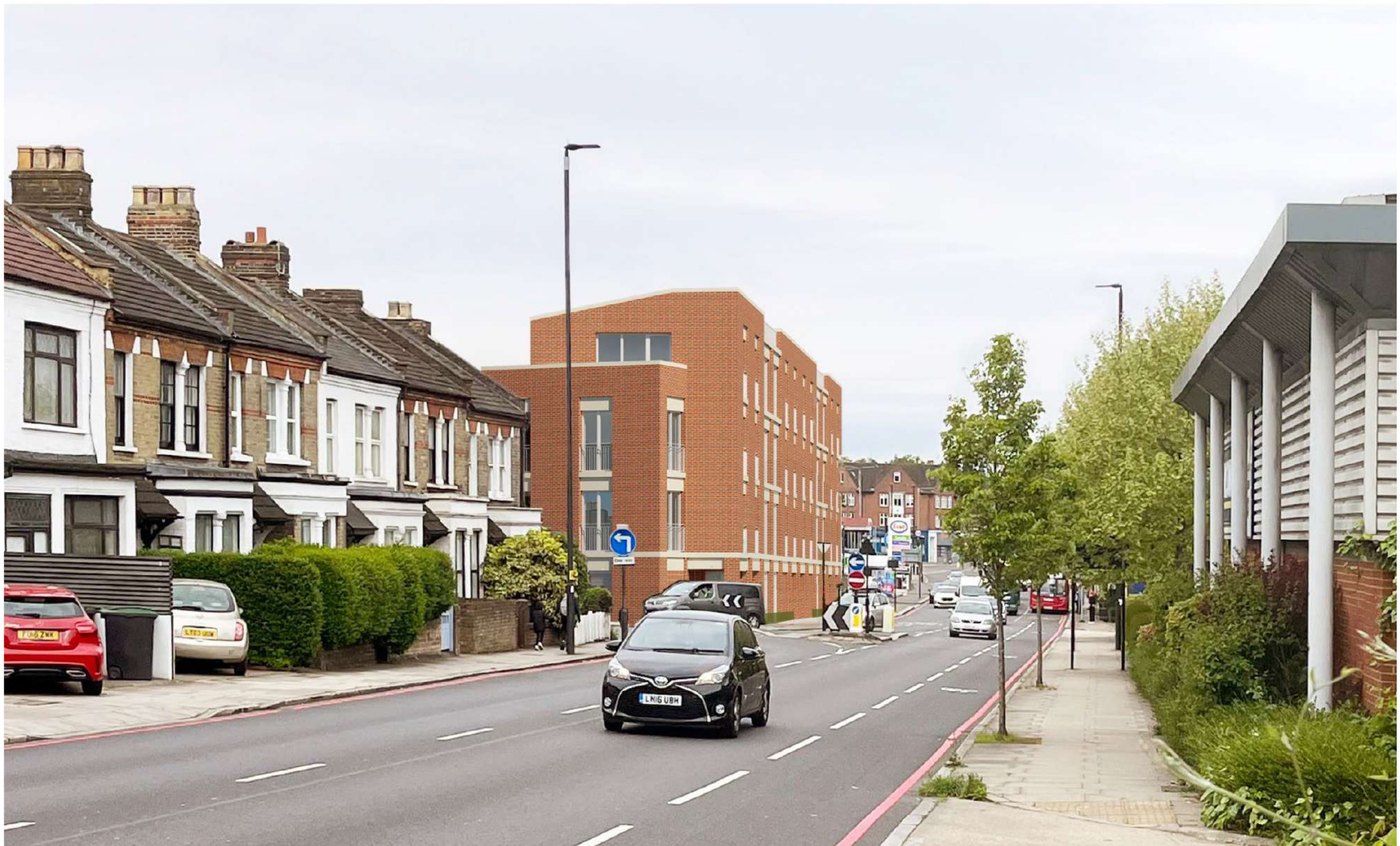
Archway Road looking North West
