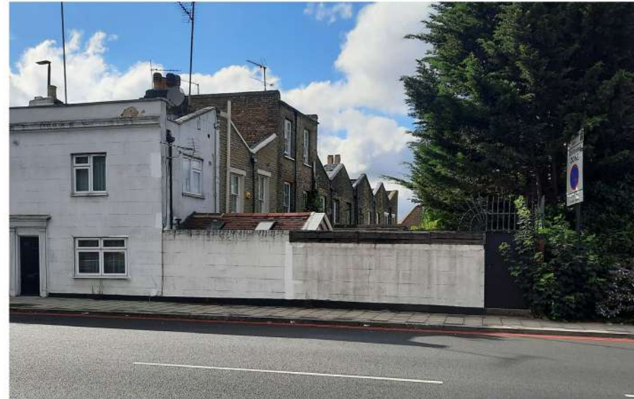
2 Rear elevation of adjacent houses and gardens from Bakers Lane
