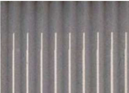
Ribbed pre-cast panels
