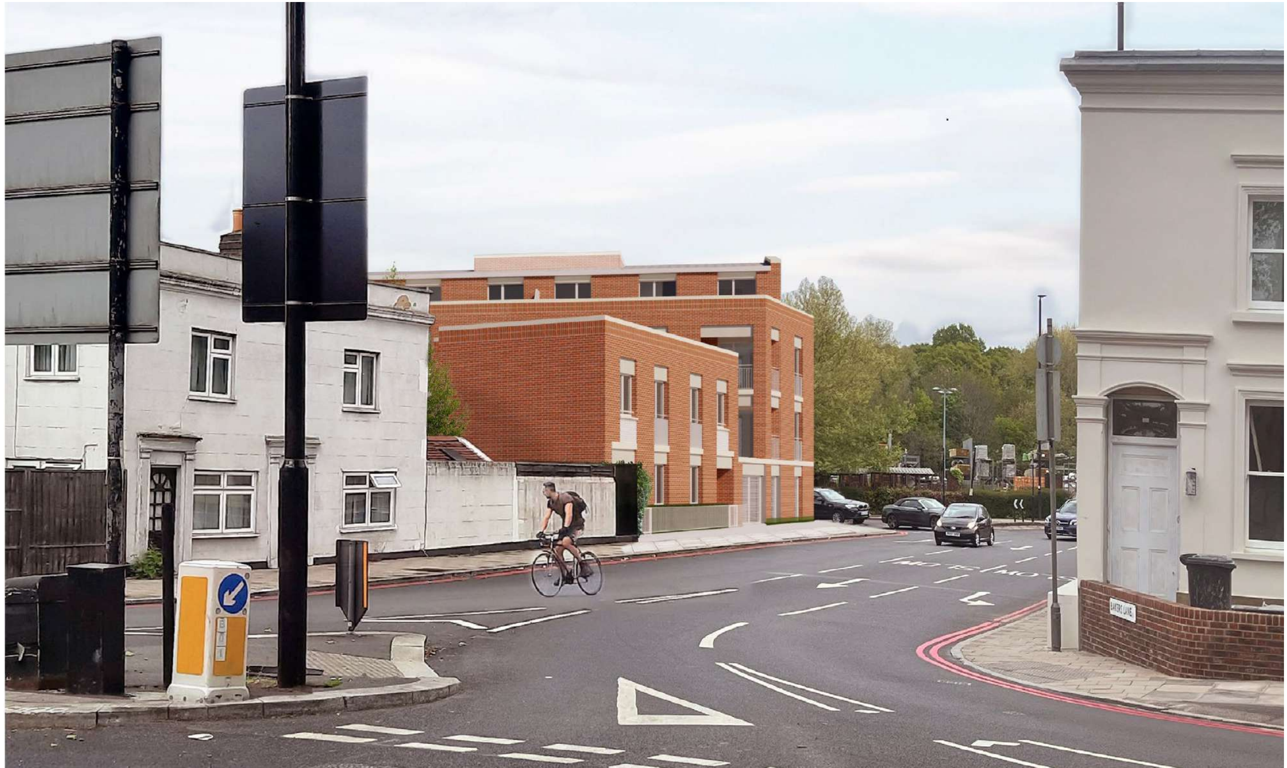
Bakers Lane looking towards Archway Road
