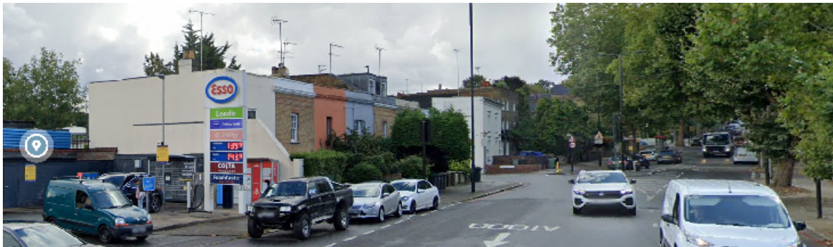
Existing view looking south-east from North Hill showing Nos. 96-108, Nos. 88 and 90 (locally listed) and Nos. 82-86 (listed Grade II) taken from Streetview, no comparative proposed view provided
