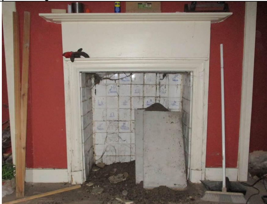
Room LG2, showing fireplace.
