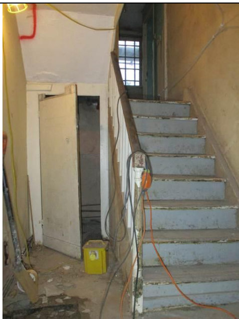
Room LG1, looking west towards staircase.
