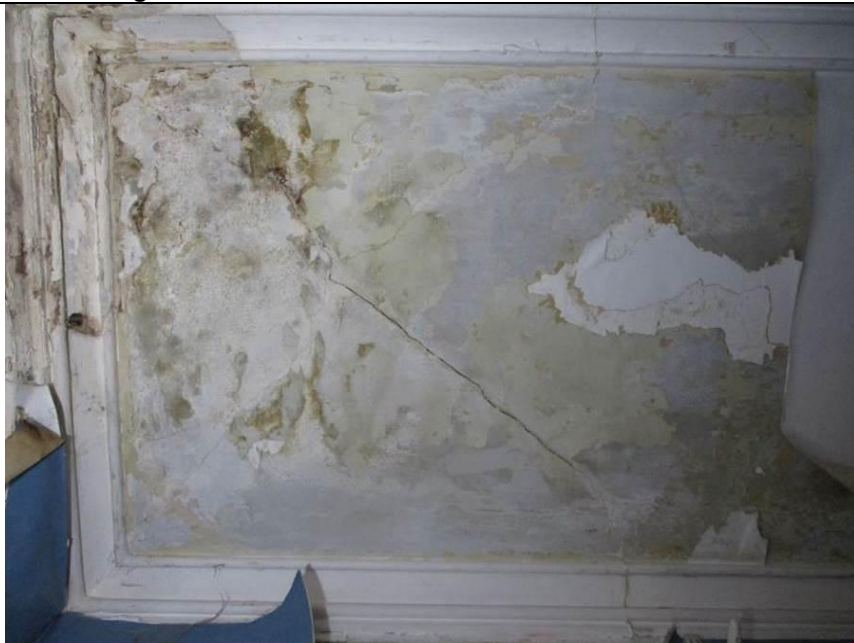
Room G1, showing plaster ceiling with cornice.
