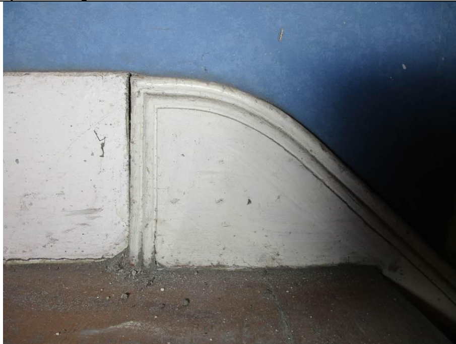
Room F1, showing the profiled staircase stringer at its junction with the adjacent plain (unprofiled) skirting.
