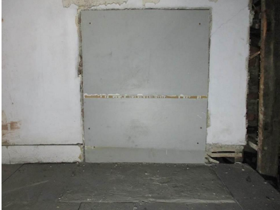
Photograph: Building Detail
