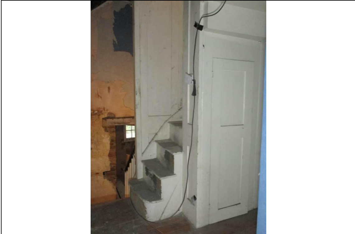
Room F1, showing the staircase between the first floor and attic (second) floor.
