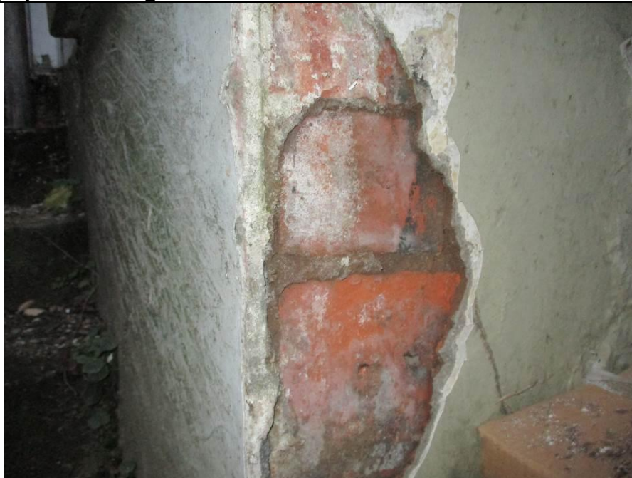
Photograph: Building Detail
