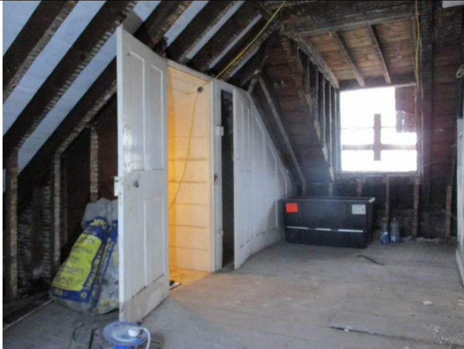
Room S1 looking west through room.
