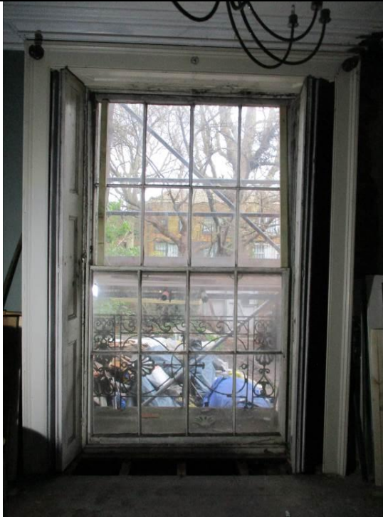
Room G2, showing window set within shutters.
