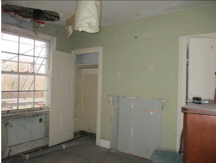
Room F3, looking northwest through room.
