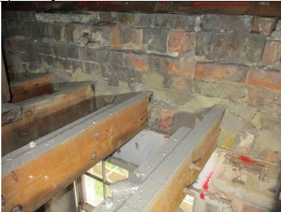
Photograph: Building Detail
