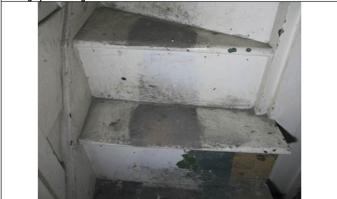
Room F1, showing the treads and risers to the staircase between first floor and attic (second) floor.
