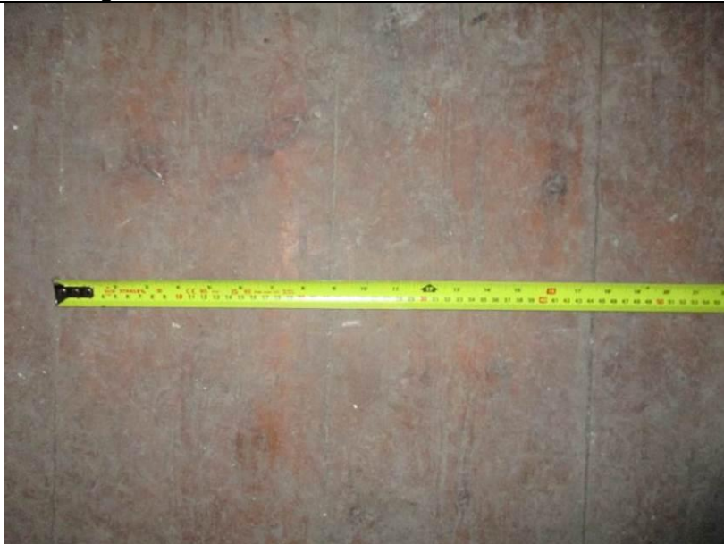
Room G3, showing floorboards.
