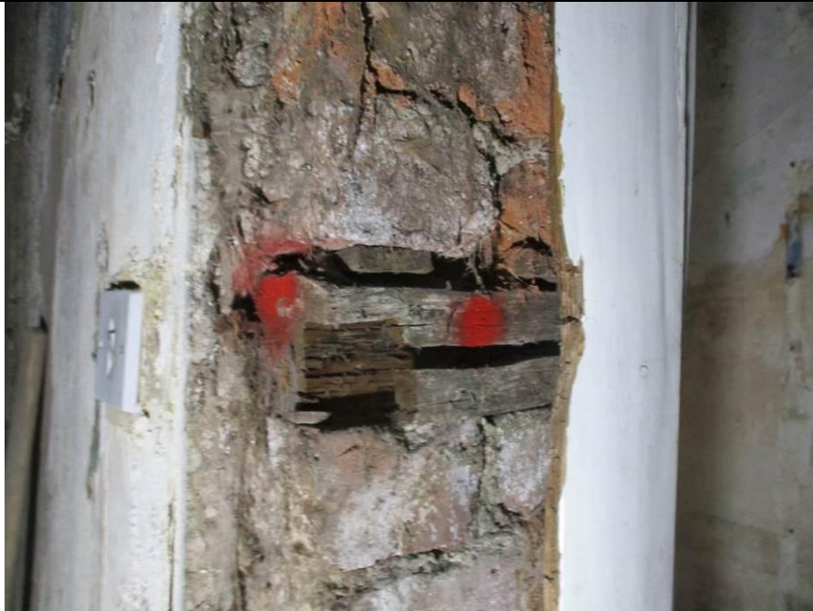
Room F2, showing timber grounds which affix doorway architrave to wall.
