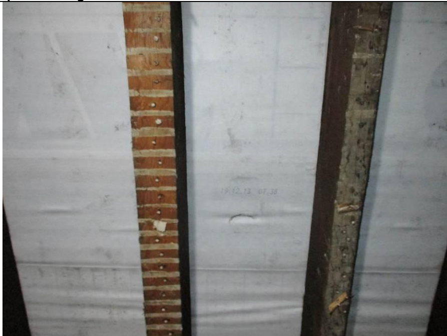
Room S1, showing the underside of south roof slope (east end) where rafters are overlaid by
