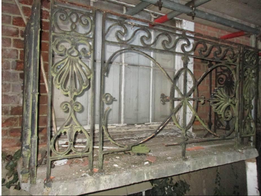
Photograph: Building Detail
