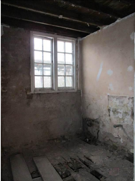
Room F4 looking west through room.
