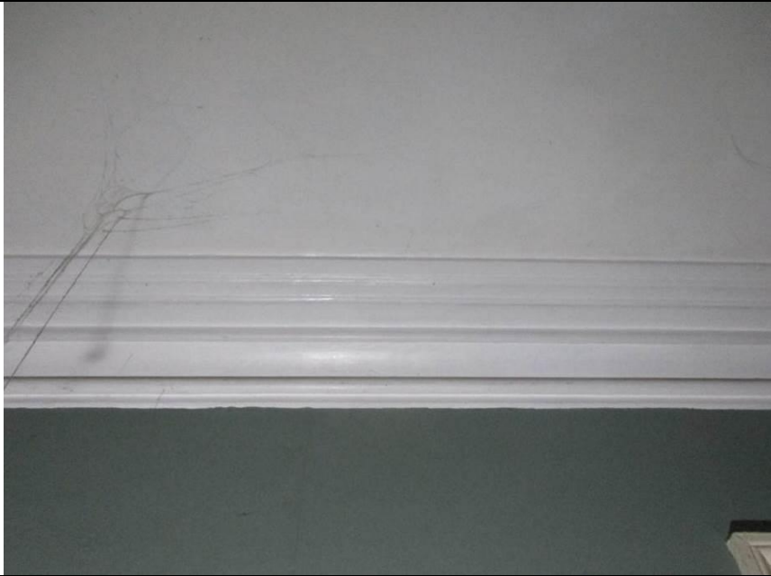
Room G2, showing cornice detail.
