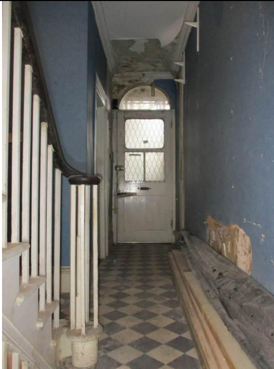
Room G1, looking east through hallway.
