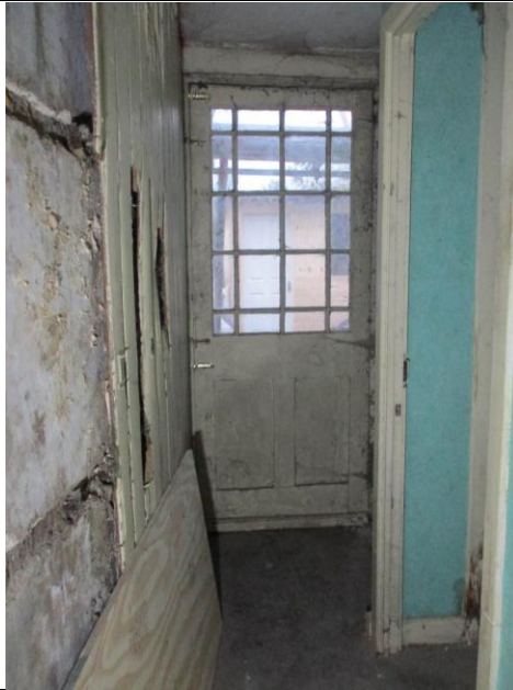
Room G4, looking west through back hallway.
