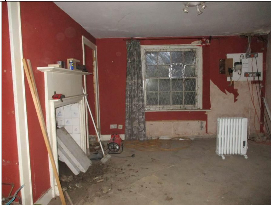
Room G1 looking east through room.
