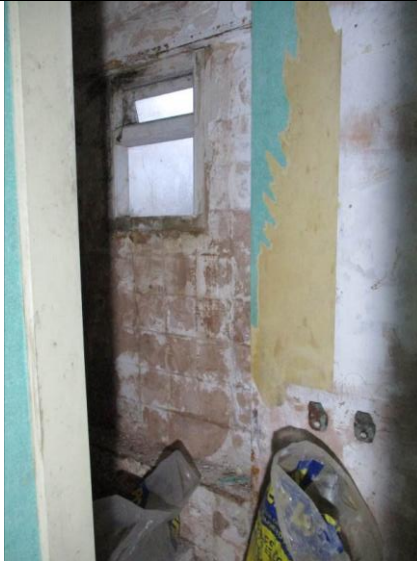
Room G5 looking into room from doorway.
