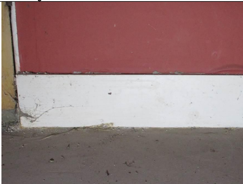
Room LG2 , showing plain skirting (without moulding).
