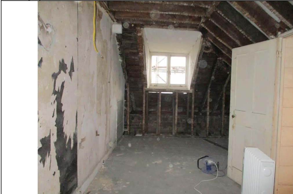
Room S1, looking east through room.
