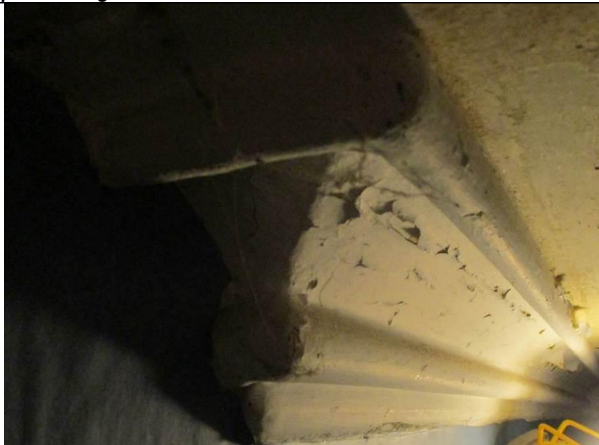
Room G1, showing cornice detail.
