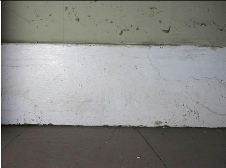
Room F3, showing skirting board.
