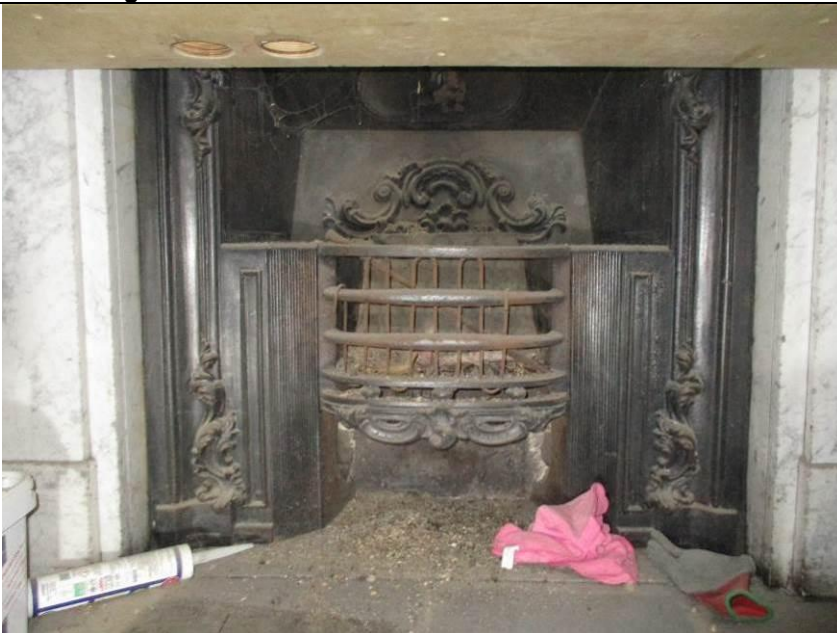
Room G2, showing cast-iron hob grate.
