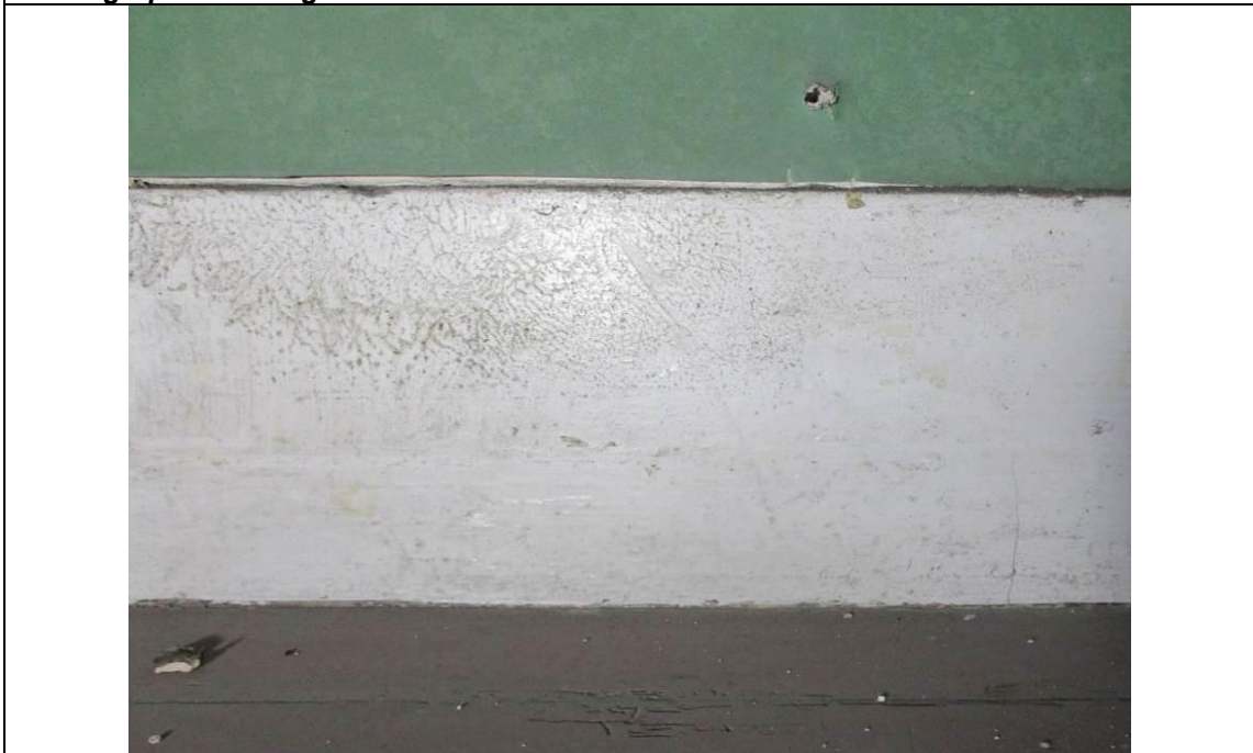
Room F2, showing skirting board detail.
