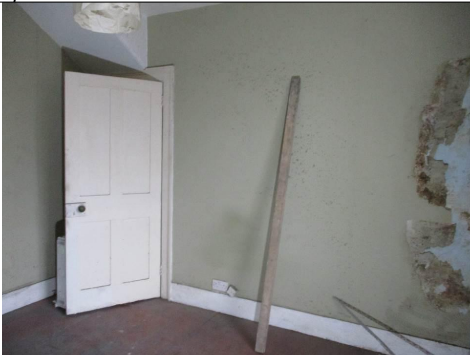
Room F3, looking southeast across room.
