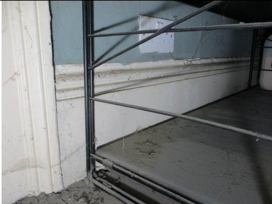
Room G3, showing skirting.
