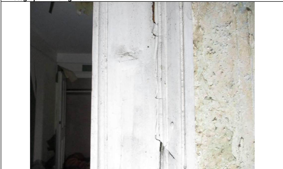
Room F1, showing the architrave detailing to the doorway into room F2. The architrave is formed of plain timber boards with applied beading.
