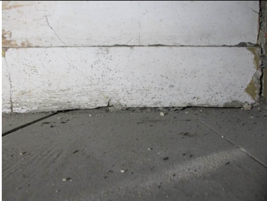
Room S1, showing plain (unprofiled) timber skirting.
