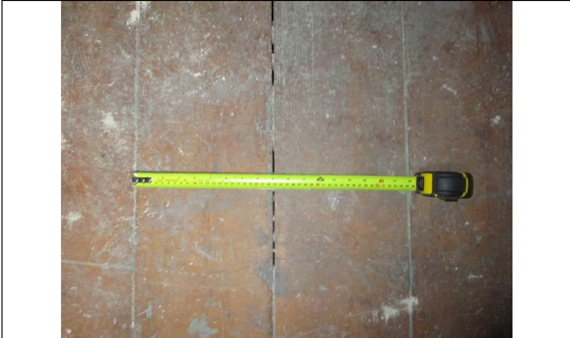
Room F1, showing floorboards. The width of the floorboards varies slightly being between 210mm-225mm (width).
