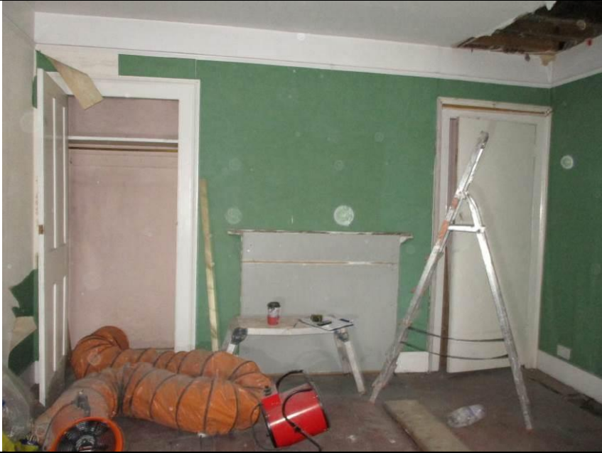
Room F2, looking north through room.
