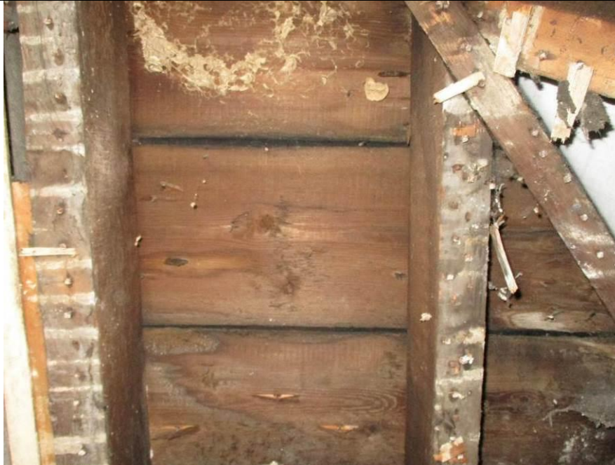
Photograph: Building Detail
