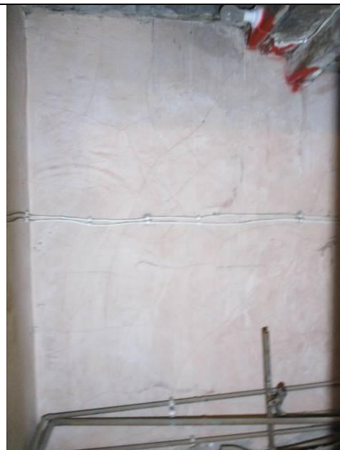
Room LG1a, looking into understairs cupboard.
