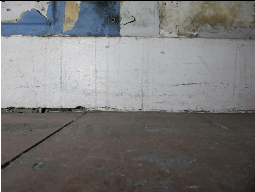
Room F1, showing skirting detail.
