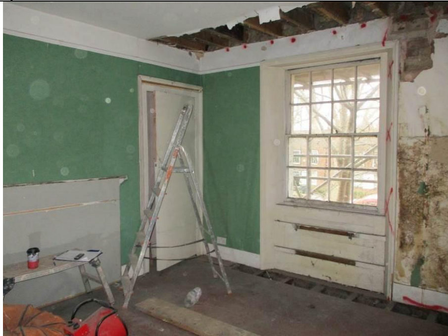
Room F2 looking west through room.
