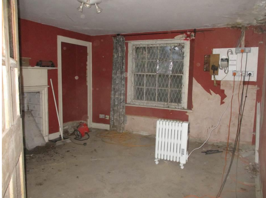
Room LG2, looking east through room.
