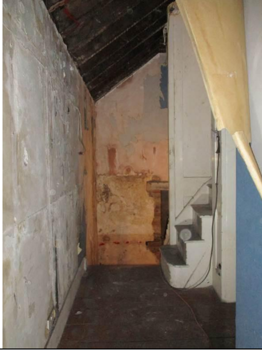
Room F1, looking west through landing.
