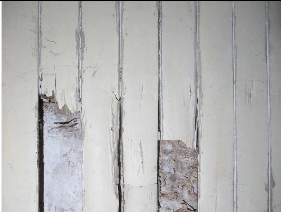
Room G4, showing wainscoting.
