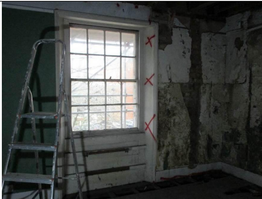
Room F2 looking east through room.
