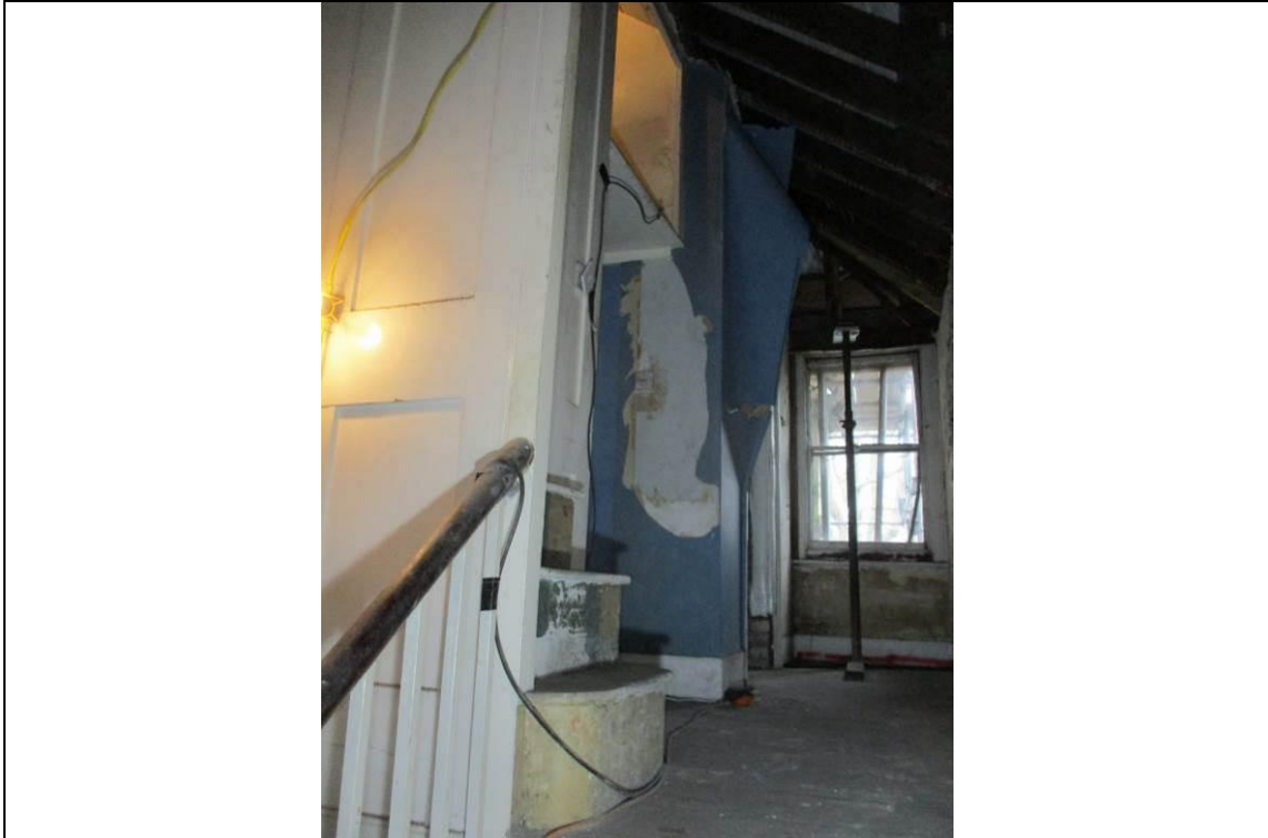
Room F1, looking east across landing.
