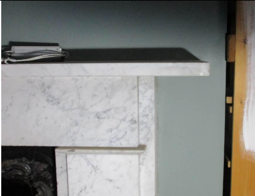
Room G2, showing detailing of marble fireplace.
