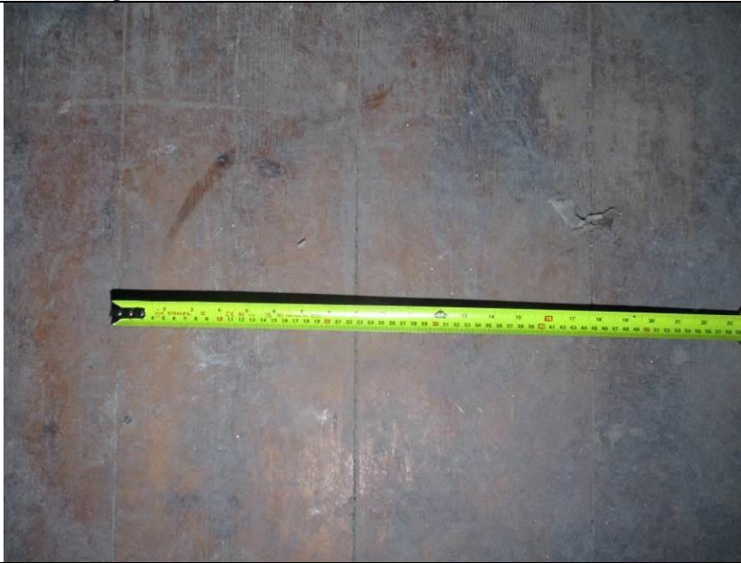
Room G2, showing floorboards.
