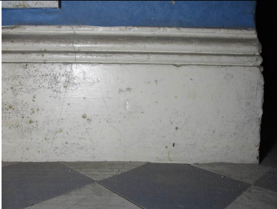
Room G1, showing profiled skirting.
