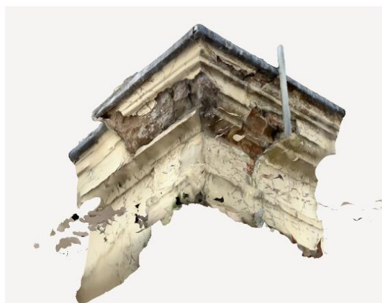
FRONT VIEW FROM CORNER BELOW
