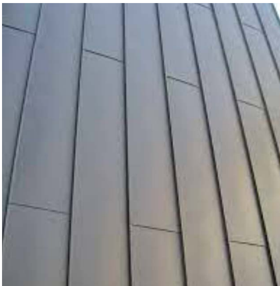
Metal cladding: Vertical standing seam zinc cladding.
