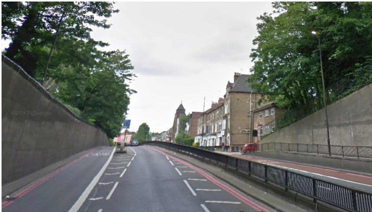
View of Archway Road on entering Highgate Conservation Area
