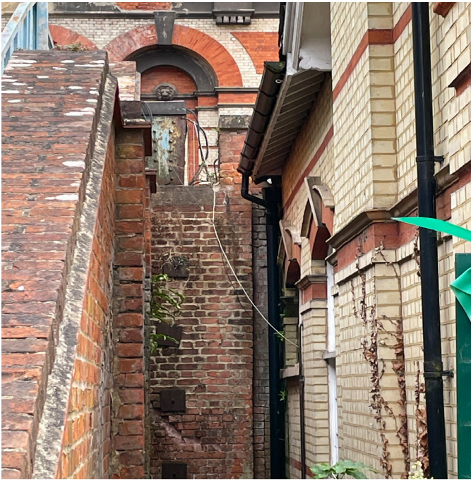
Like-for-like repairs to Southern brick wall adjacent to the 'CUFOS' building
