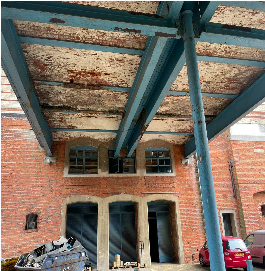
Like-for-like repairs/replacement to vaulted arch brickwork
