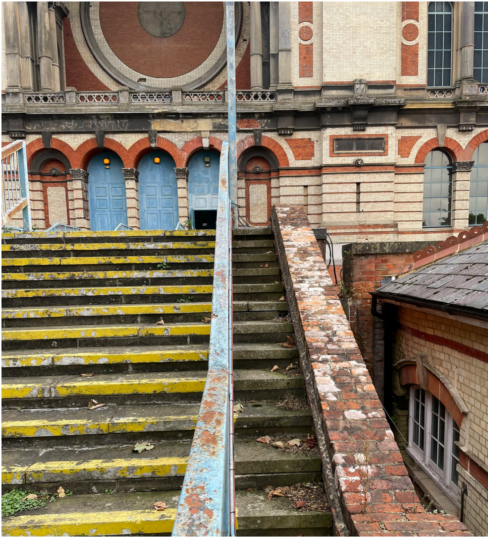
Like-for-like repair/replacement of stone steps.
