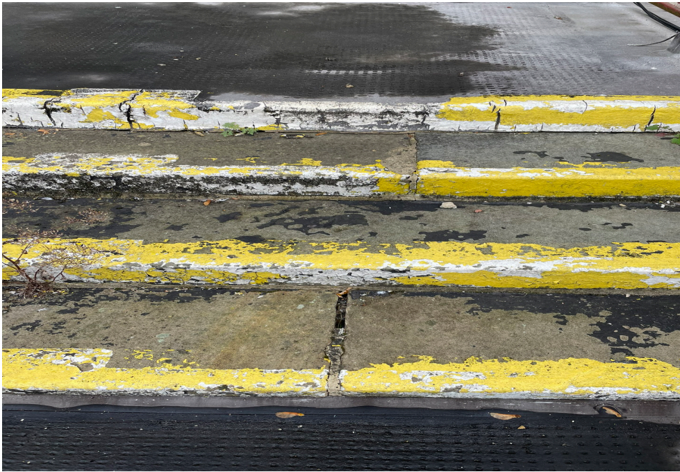
New like-for-like riser stone step to achieve new drainage falls
