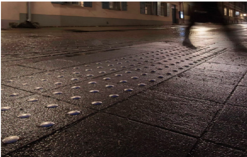
Blister surface studs - alternative to corduroy strips
