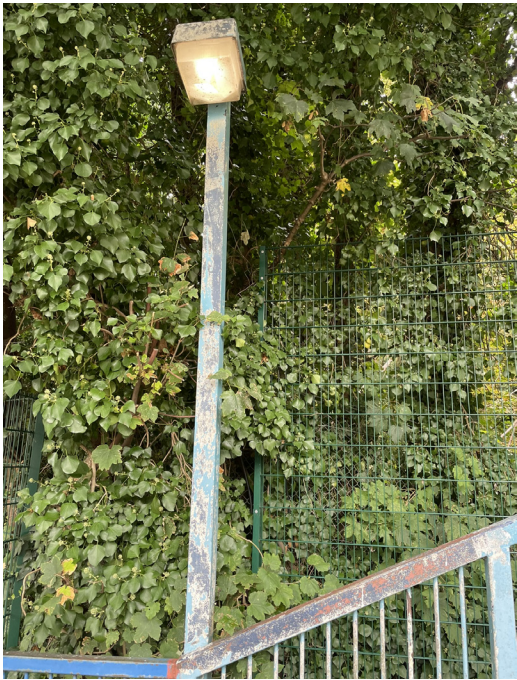
Like-for-like replacement to lights
