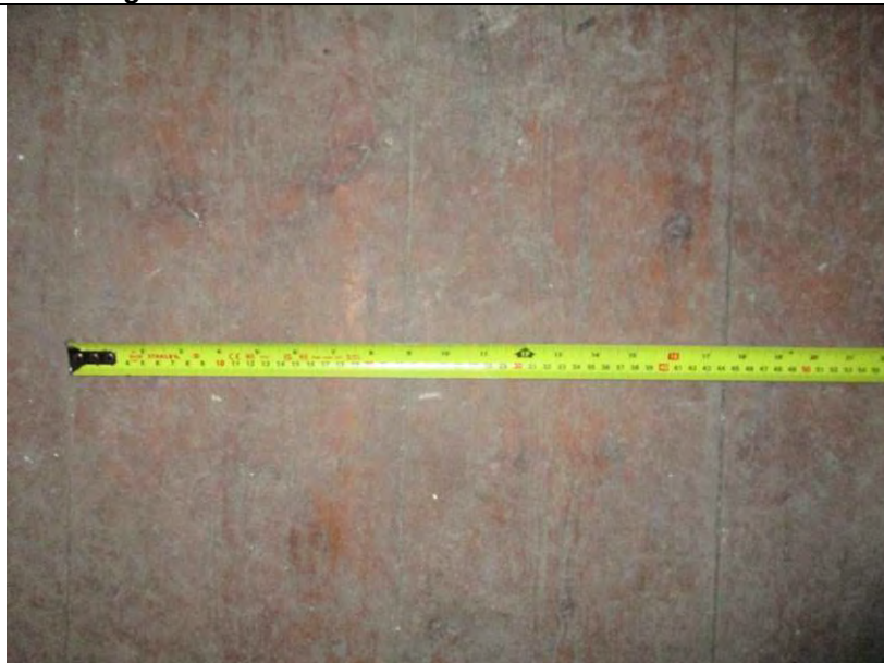
Room G3, showing floorboards.
