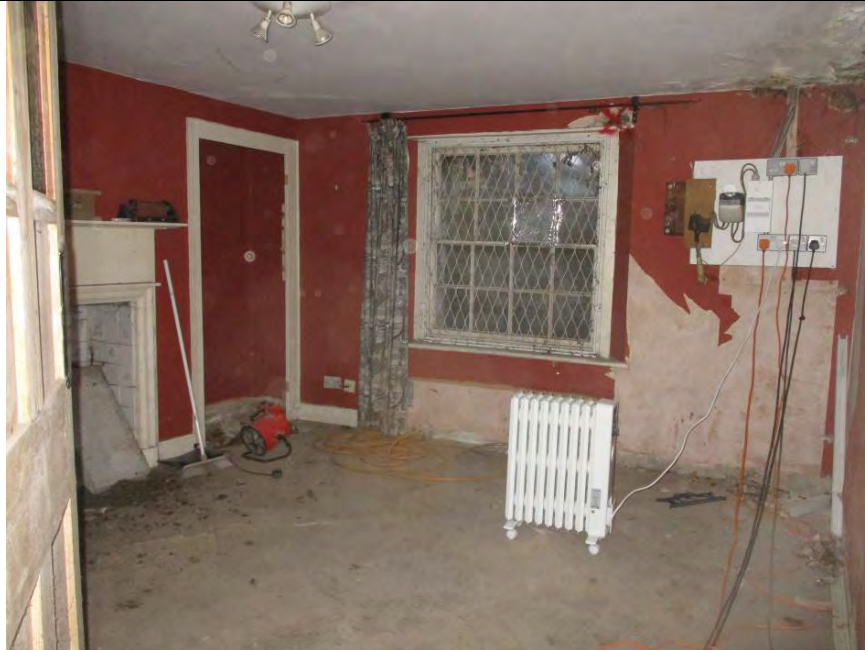
Room LG2, looking east through room.
