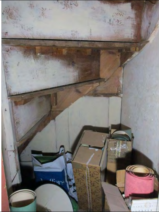
Room F1a, the cupboard under the staircase.
