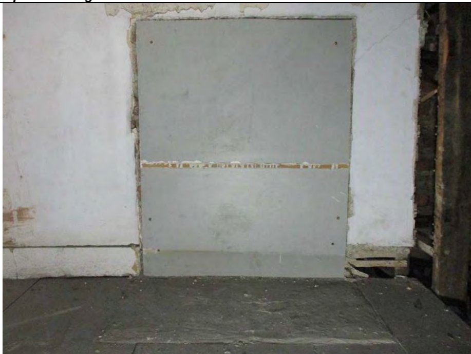
Room S1, showing the position of former fireplace within north party wall. The fireplace (surround and grate) has previously been removed although the hearth remains within the floor.
