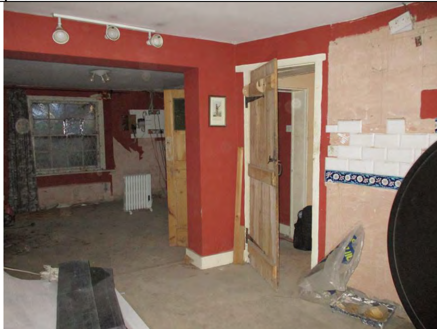
Room LG3, looking southeast through room.
