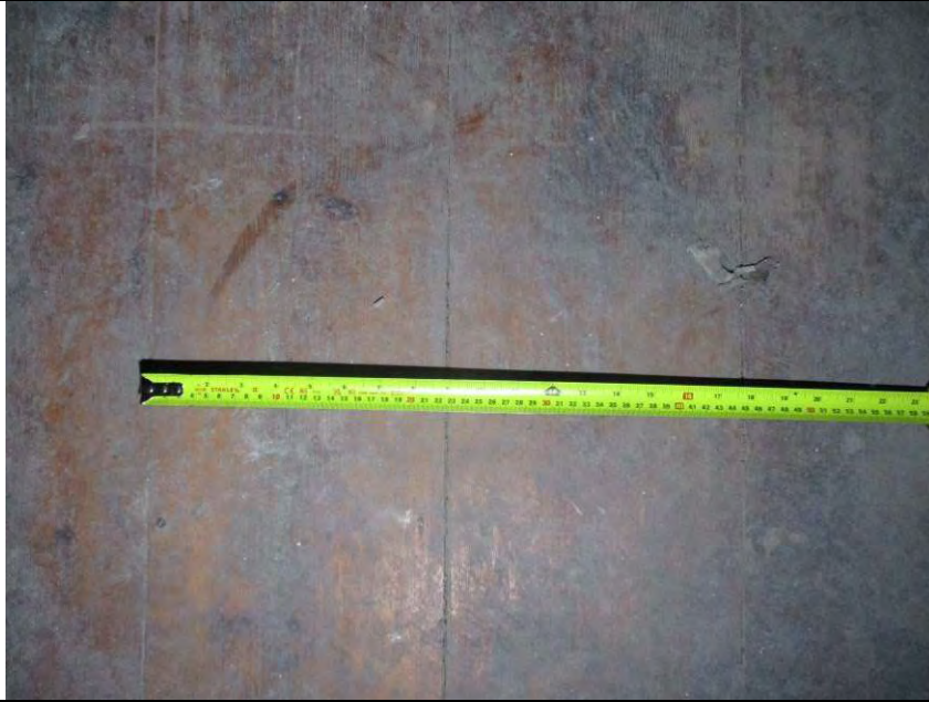
Room G2, showing floorboards.
