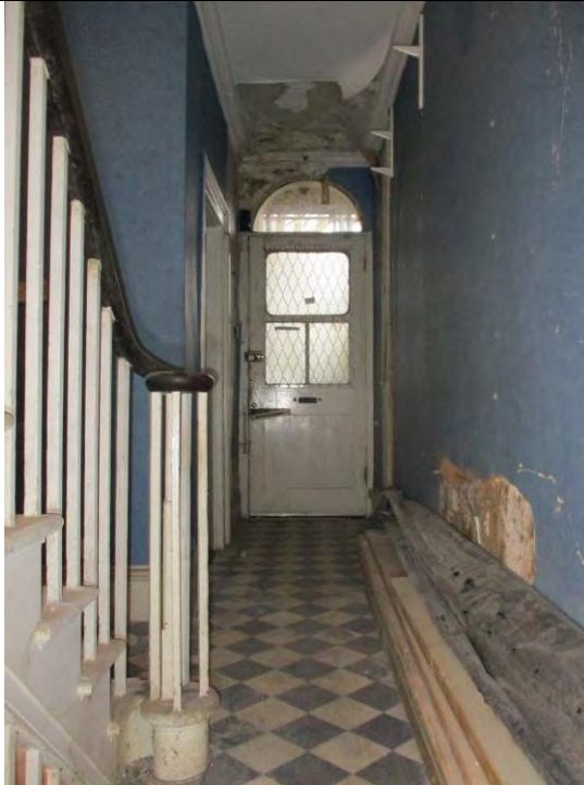
Room G1, looking east through hallway.
