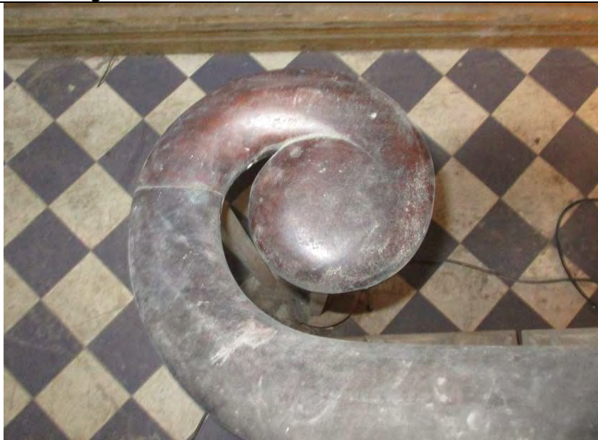
Room G1, showing the handrail detail at the curtail step.
