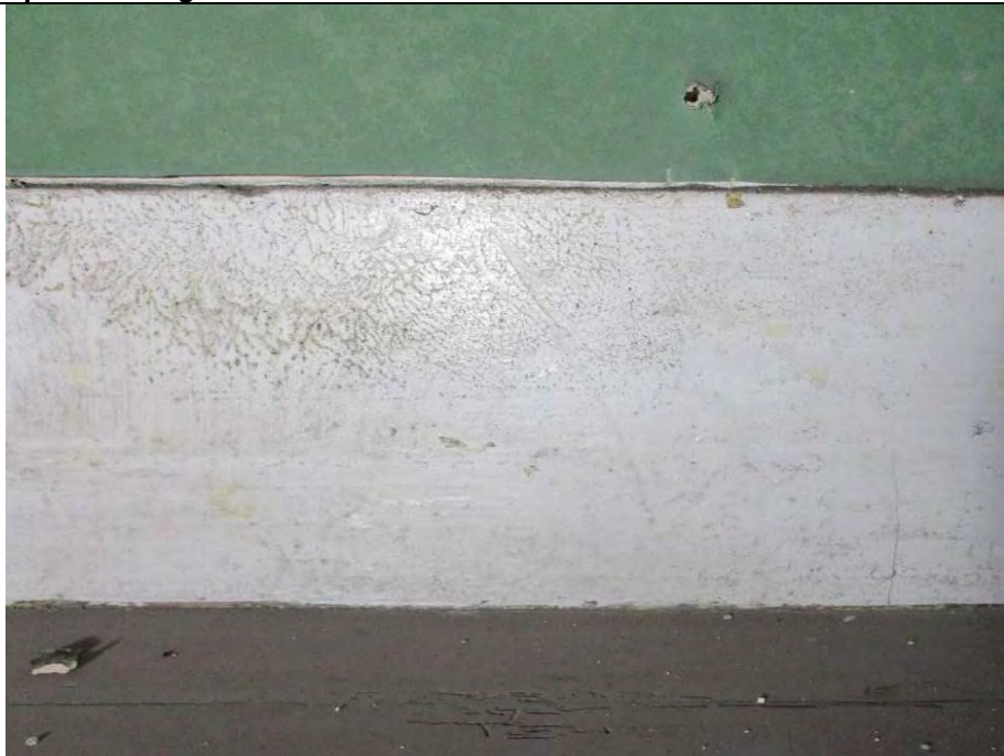
Room F2, showing skirting board detail.
