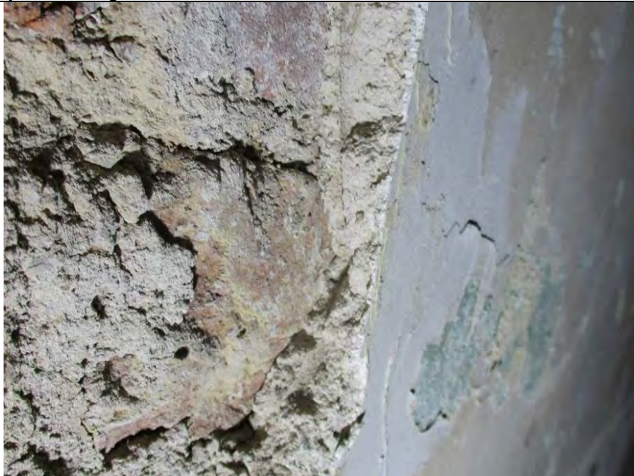
Room F1, showing the south wall which comprises of a plaster finish onto brickwork. The plaster finish comprises of a two-coat plaster - scratch coat and finish coat.
