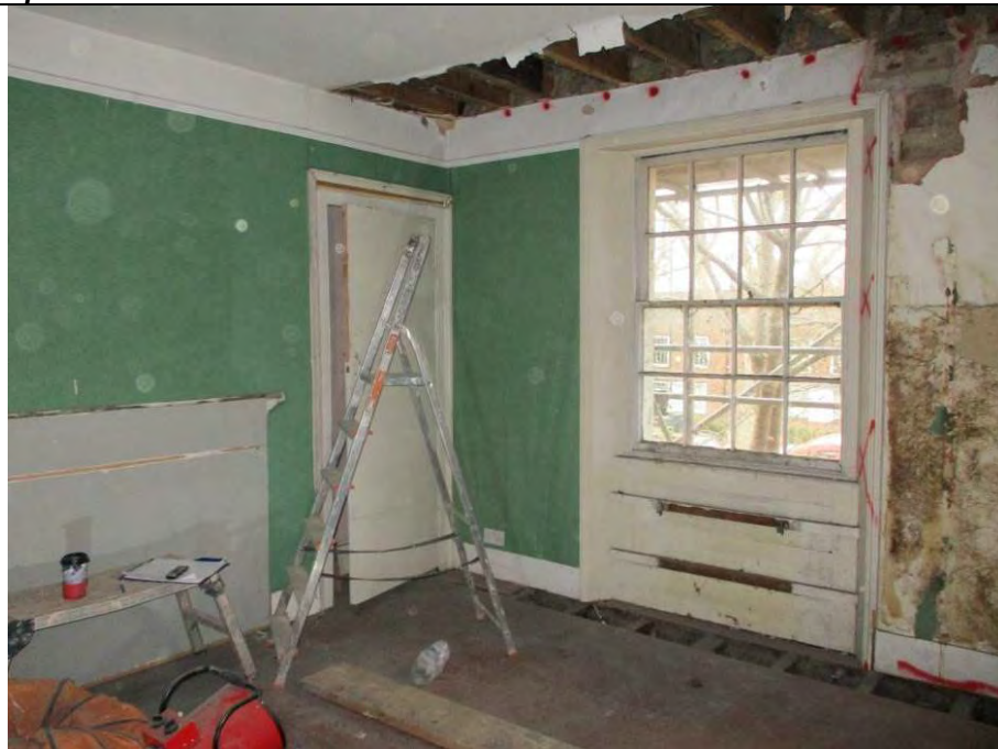
Room F2 looking west through room.
