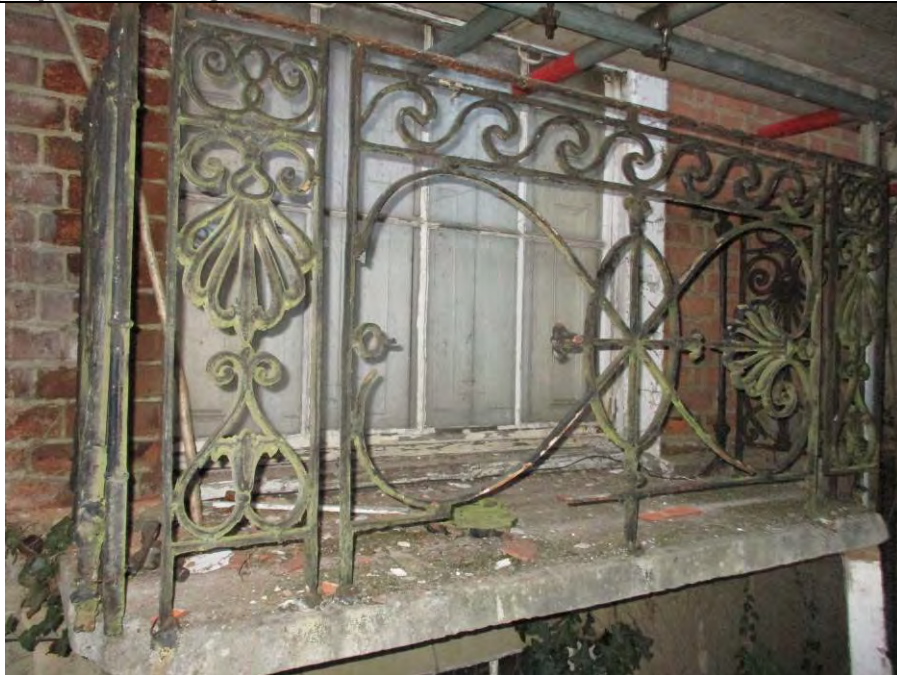
Front elevation, showing metal balconette to ground floor window.
