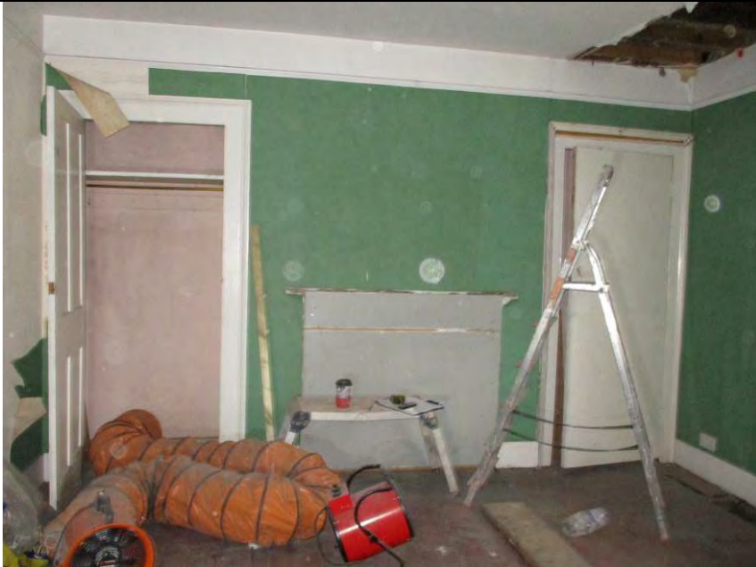
Room F2, looking north through room.
