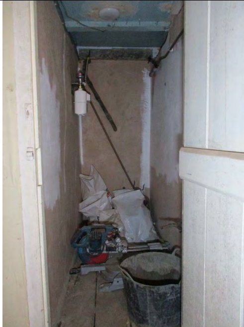
Room LG1b, showing the cupboard with undecorated gypsum plaster wall finishes.
