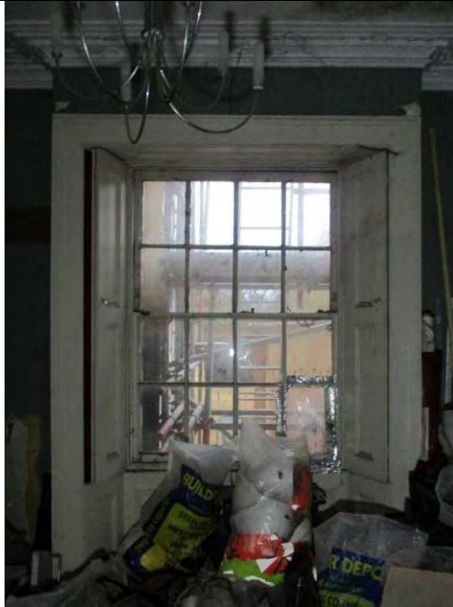
Room G3, showing window with splayed reveal and shutters.
