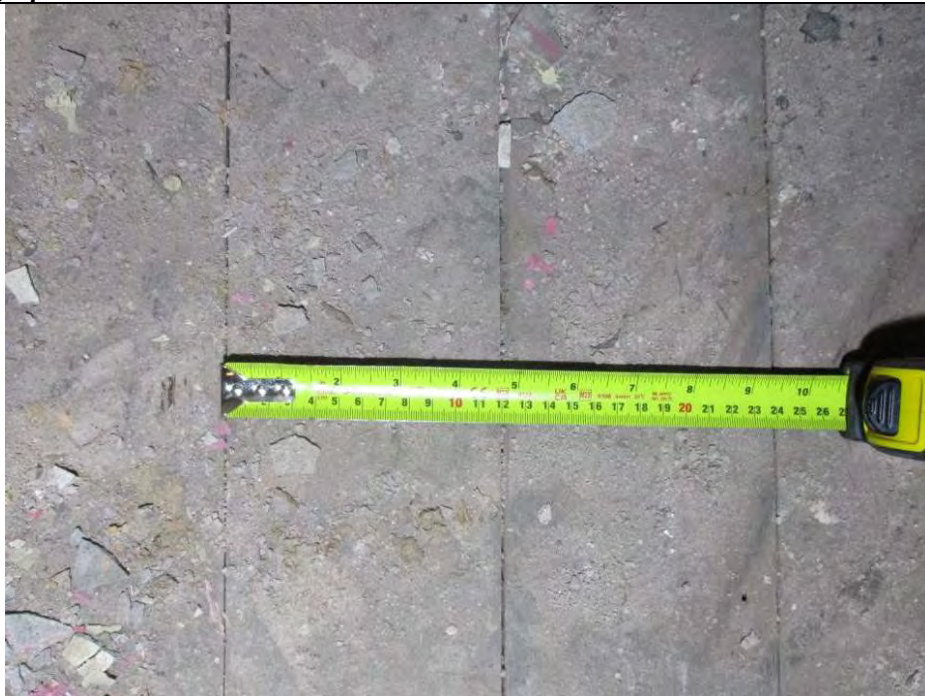
Room F4, showing floorboards.
