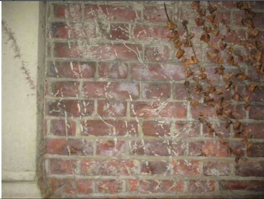
Front elevation, showing red brick laid to a bastardized Flemish bond with later cement repointing.
