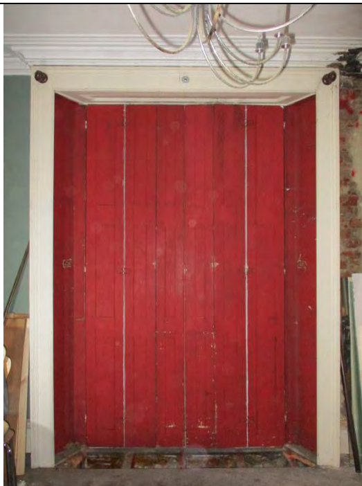
Room G2, showing panelled shutters to window.
