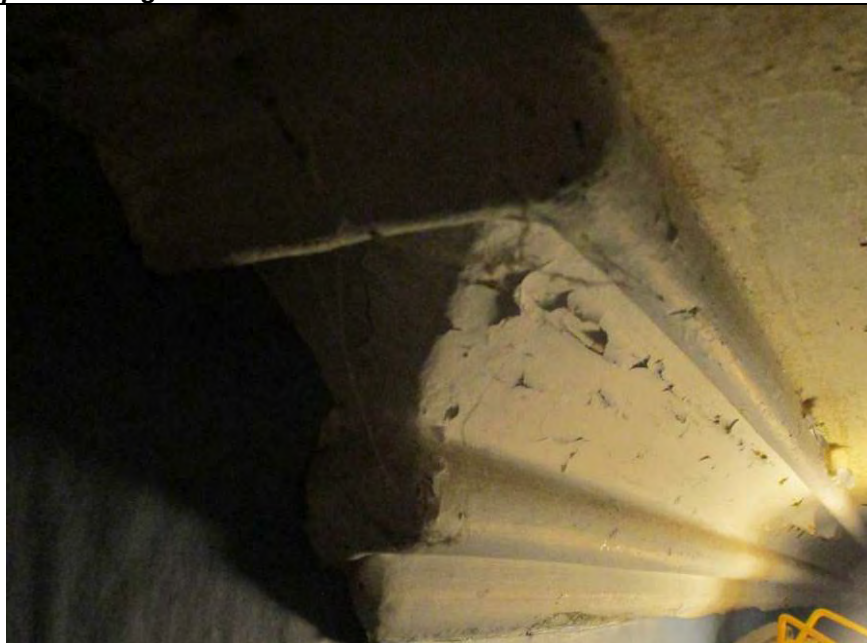
Room G1, showing cornice detail.
