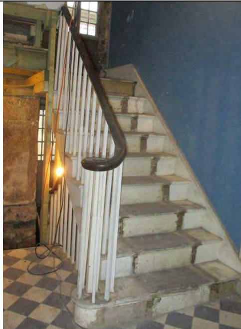
Room G1, showing staircase with curtail step to bottom of stair.
