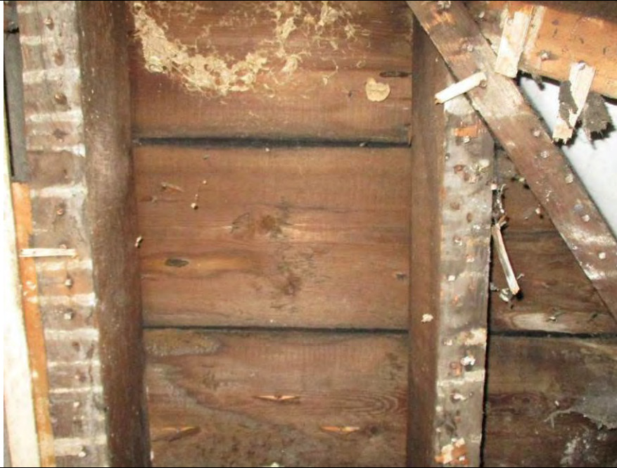
Room S1, showing the underside of the west roof slope with rafters are overlaid by sarking boards which are overlaid by roofing felt.
