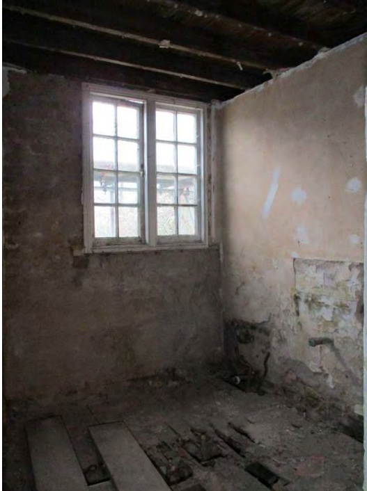
Room F4 looking west through room.
