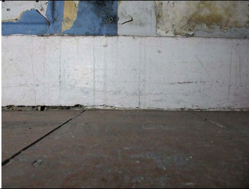
Room F1, showing skirting detail.
