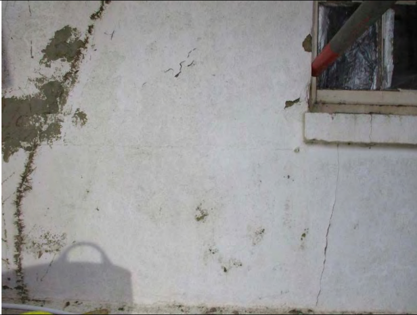
Rear (west) elevation. Painted render (assumed over brickwork). The faint lines of an incised detailing are visible within the render finish.
