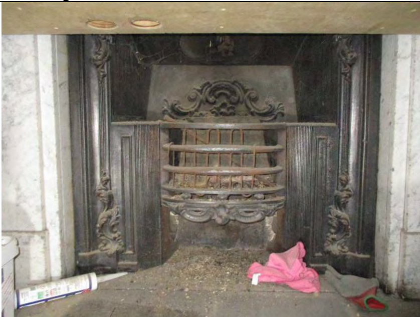
Room G2, showing cast-iron hob grate.
