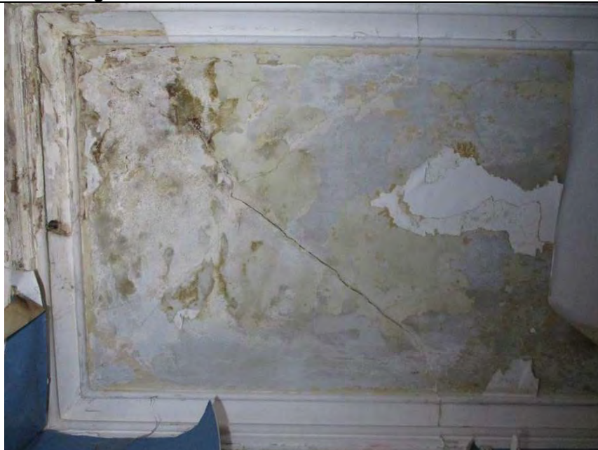
Room G1, showing plaster ceiling with cornice.
