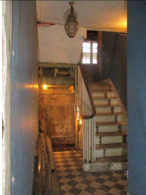
Room G1 looking west through hallway.
