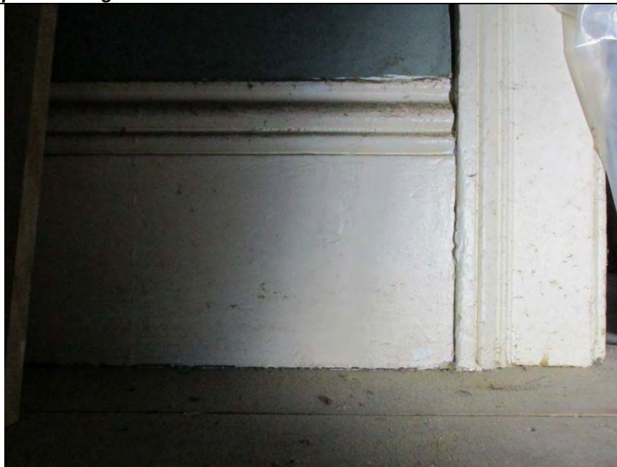
Room G2, showing the profiled skirting boards.
