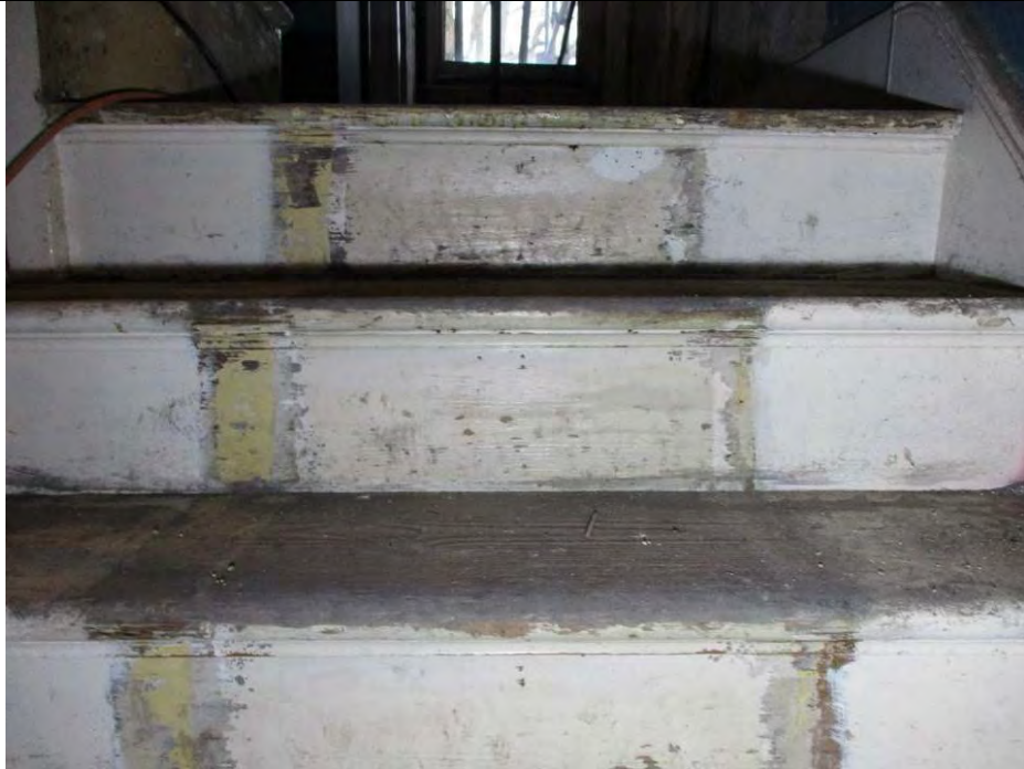
Room F1, showing the treads and risers to the staircase.
