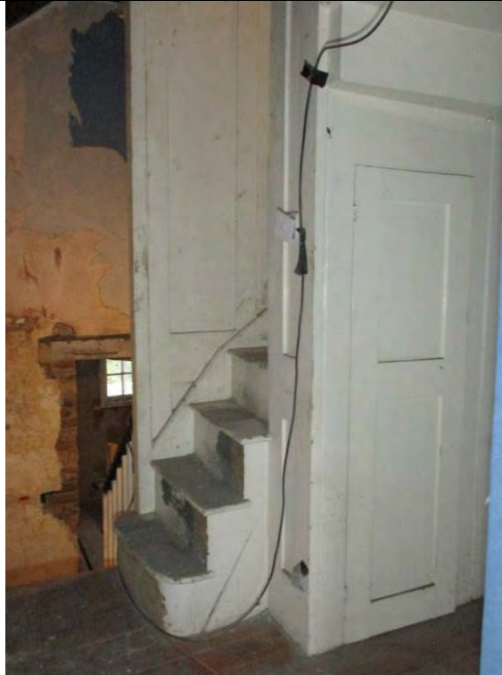
Room F1, showing the staircase between the first floor and attic (second) floor.
