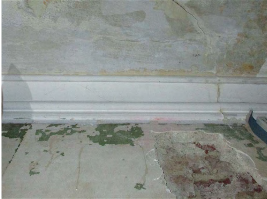
Room G1, showing cornice detail.
