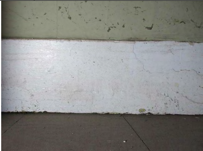
Room F3, showing skirting board.
