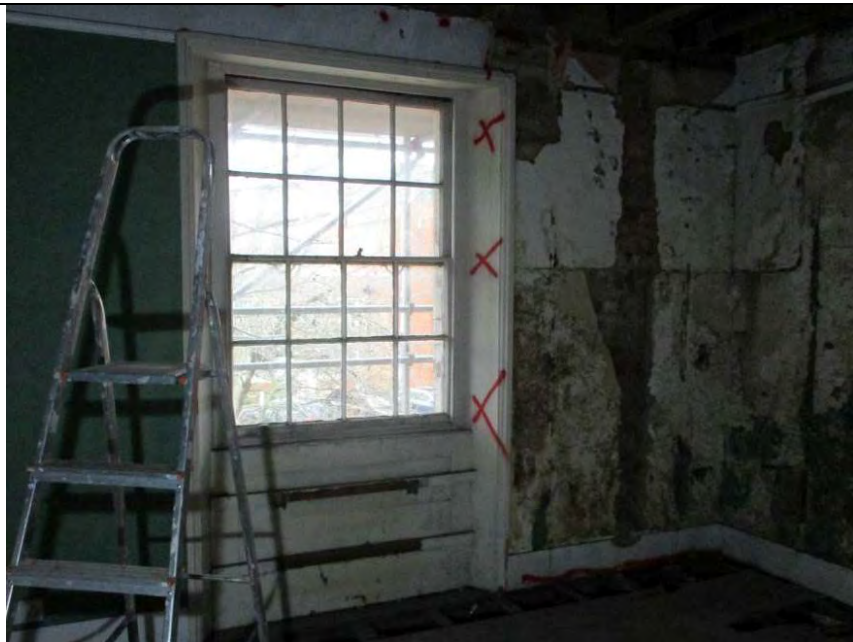
Room F2 looking east through room.
