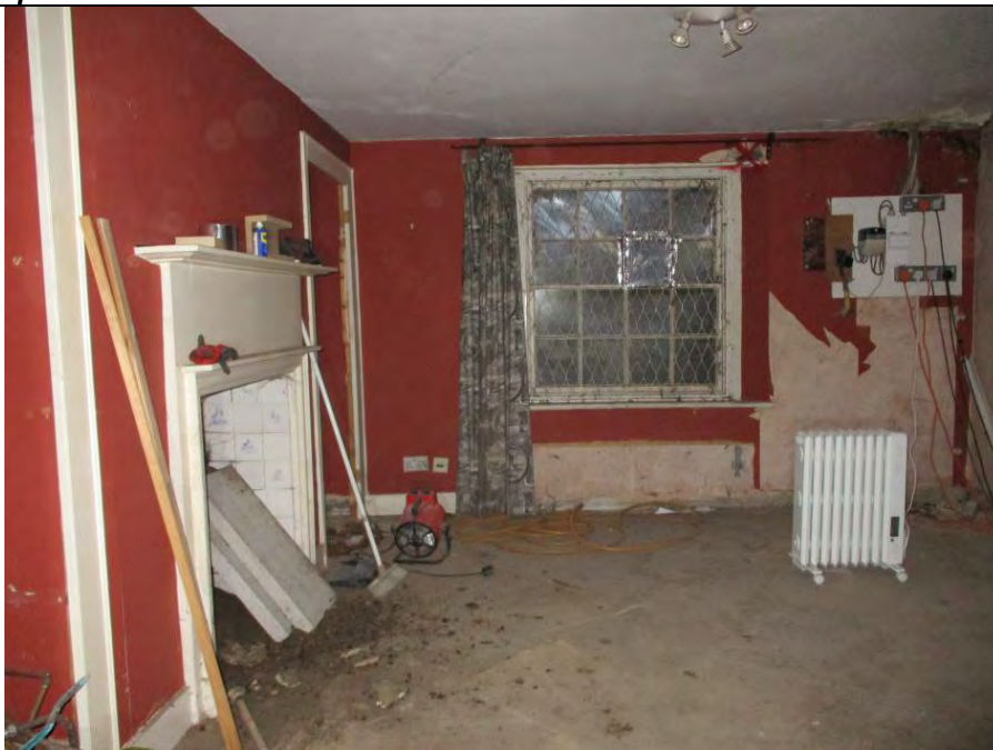
Room G1 looking east through room.
