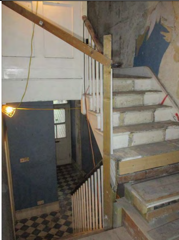
Room F1, showing the dogleg staircase of open string construction from the half landing up to the first floor.
