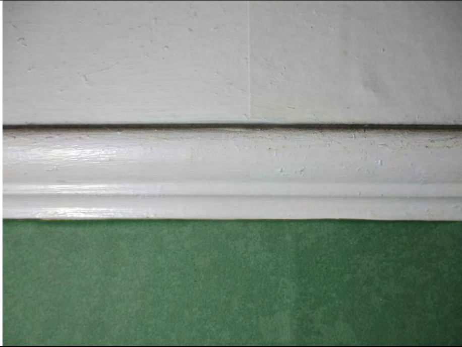
Room F2, showing picture rail detail.
