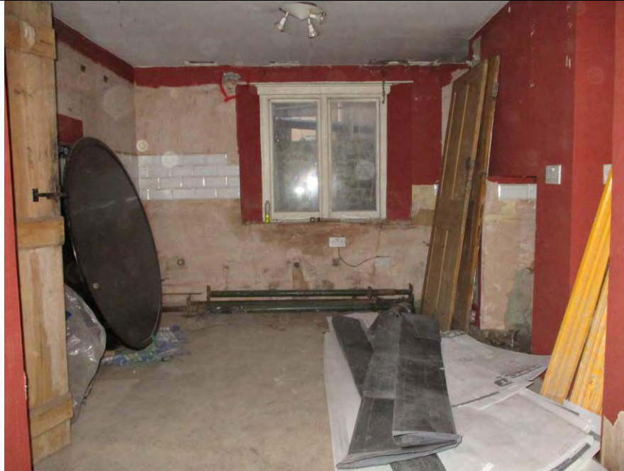
Room LG3, looking west through room.
