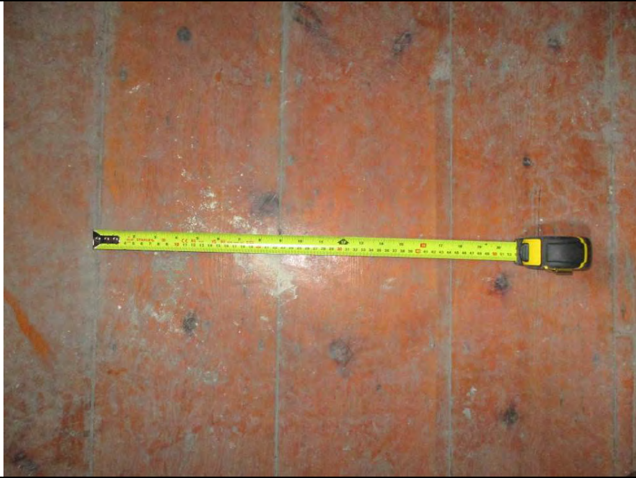
Room F3, showing floorboards
