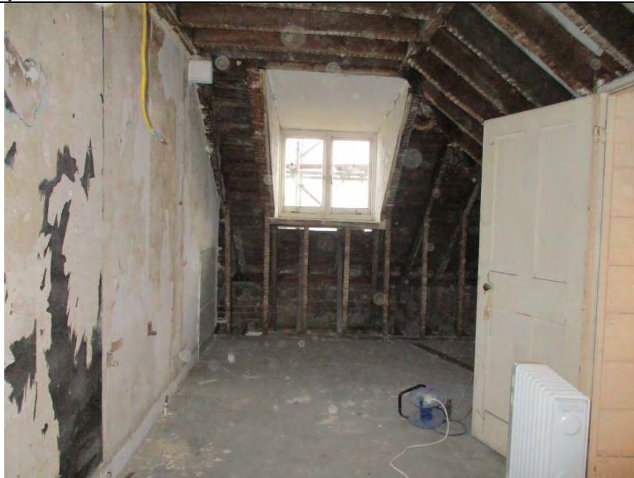
Room S1, looking east through room.
