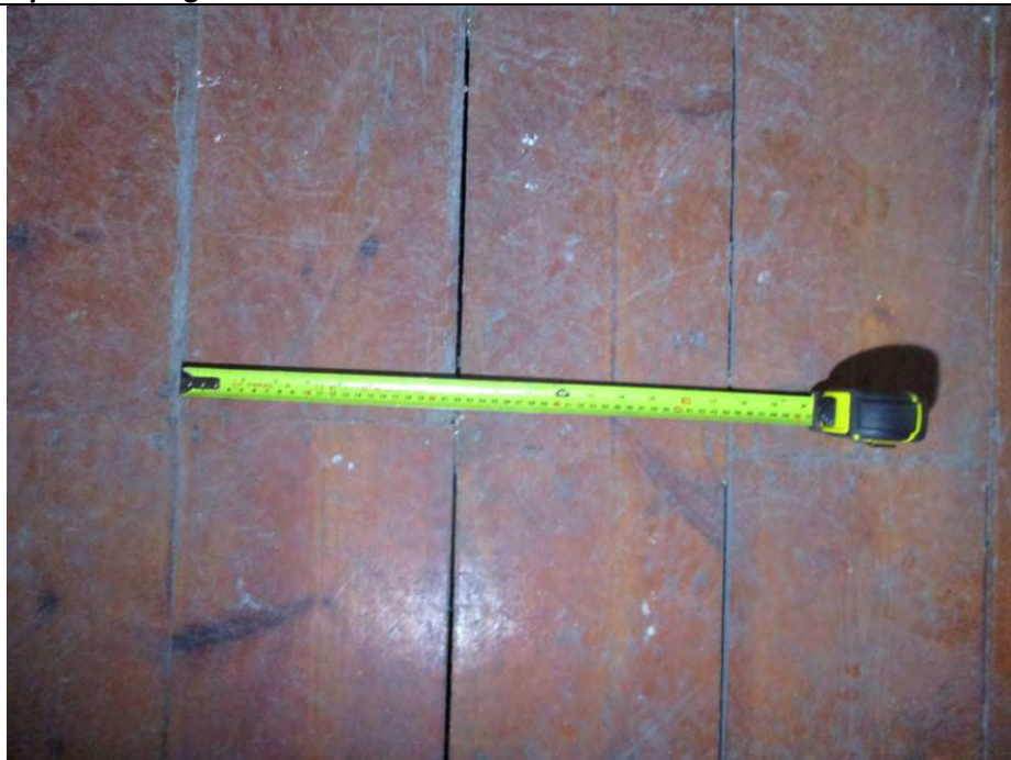
Room F2, showing floorboards.
