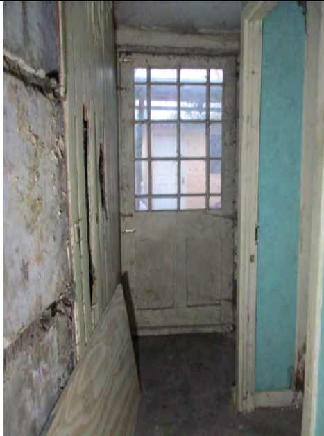
Room G4, looking west through back hallway.
