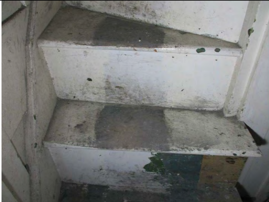
Room F1, showing the treads and risers to the staircase between first floor and attic (second) floor.
