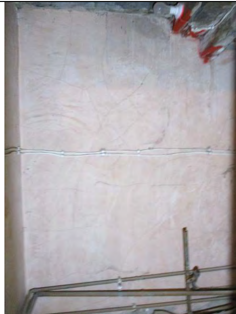
Room LG1a, looking into understairs cupboard.
