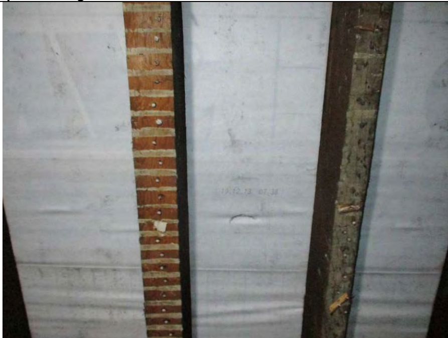
Room S1, showing the underside of south roof slope (east end) where rafters are overlaid by an assume breather membrane with production date stamp 19/12/13.
