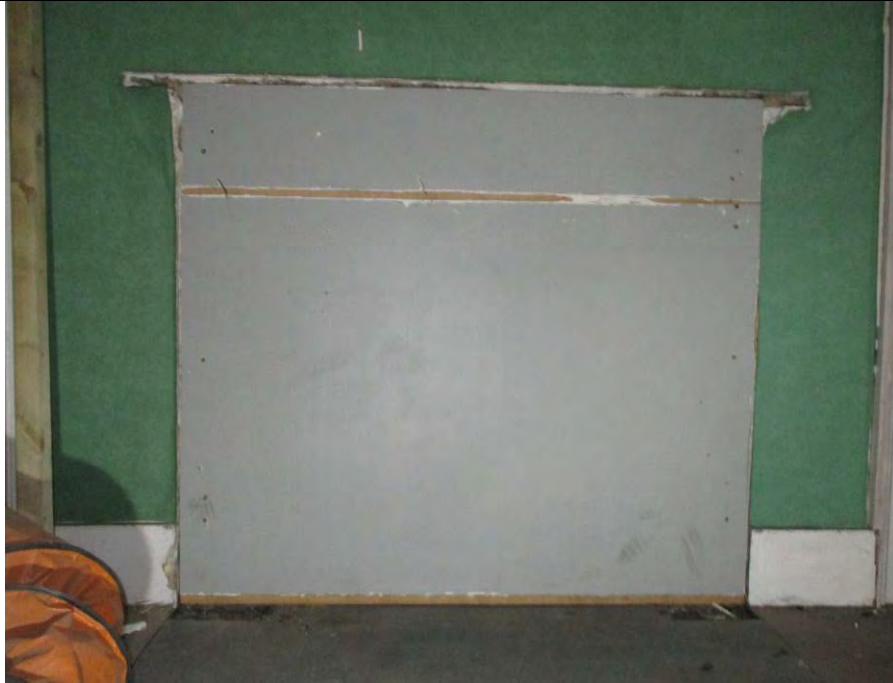
Room F2, showing location of former fireplace.
