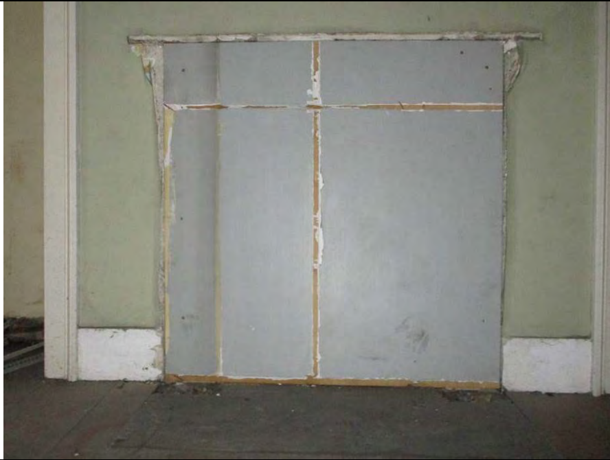
Room F3, showing location of former fireplace.
