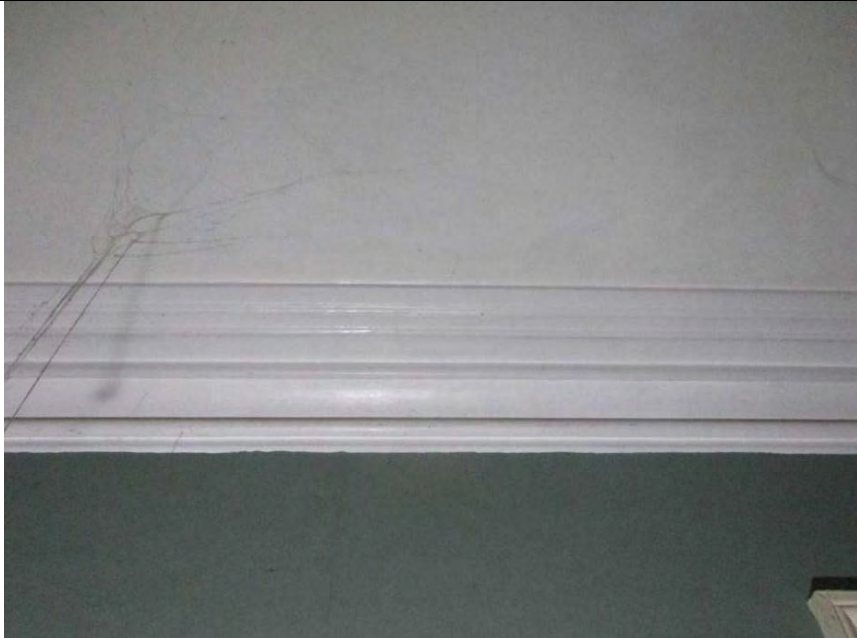
Room G2, showing cornice detail.
