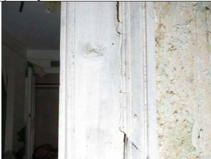
Room F1, showing the architrave detailing to the doorway into room F2. The architrave is formed of plain timber boards with applied beading.
