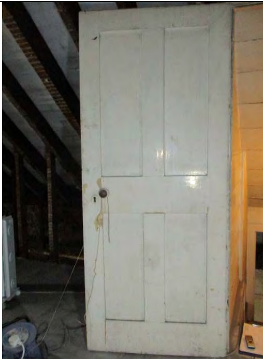
Room S1, showing four-panel internal door with key plate and handle to outer side of door.
