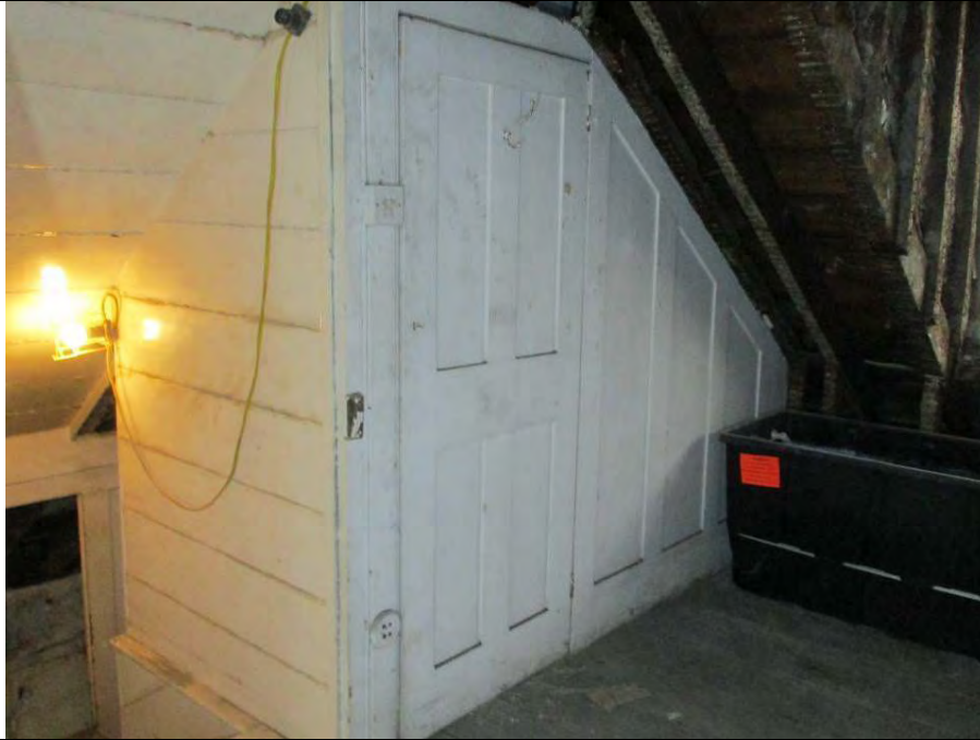
Room S1, showing room S1a as a timber built-in cupboard within the southwest corner of room.
