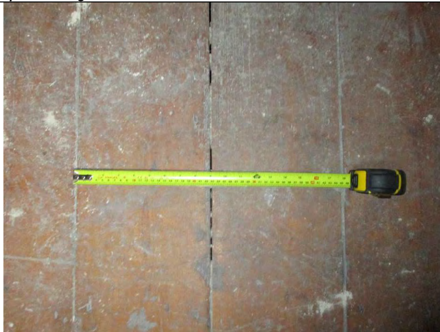
Room F1, showing floorboards. The width of the floorboards varies slightly being between 210mm-225mm (width).
