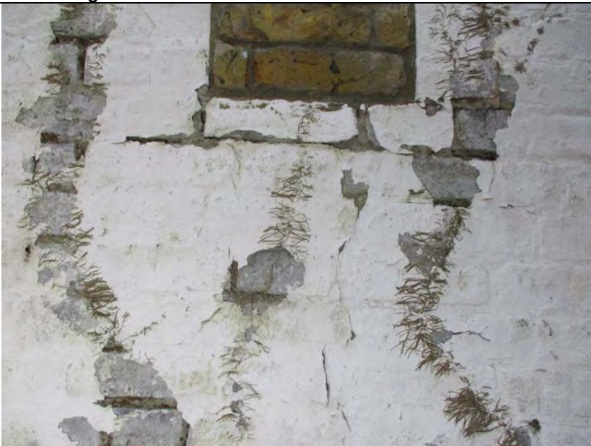
Rear (west) elevation showing the painted brickwork of the flat roof addition.
