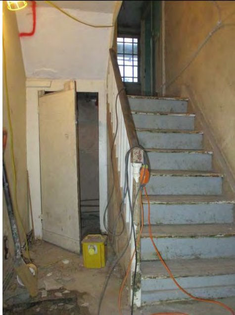
Room LG1, looking west towards staircase.
