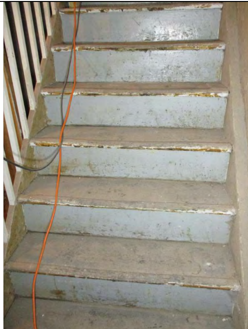
Room LG1, showing staircase (lower flight) between ground floor and lower ground floor.
