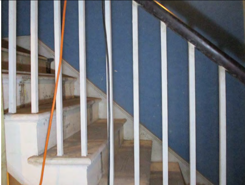
Room G1, showing open string staircase with stick spindles.
