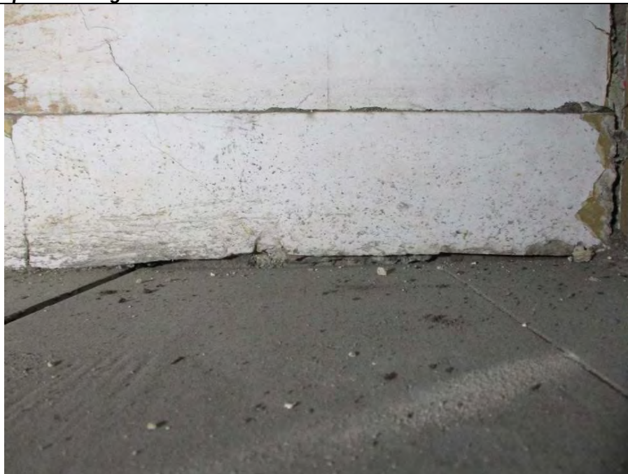
Room S1, showing plain (unprofiled) timber skirting.
