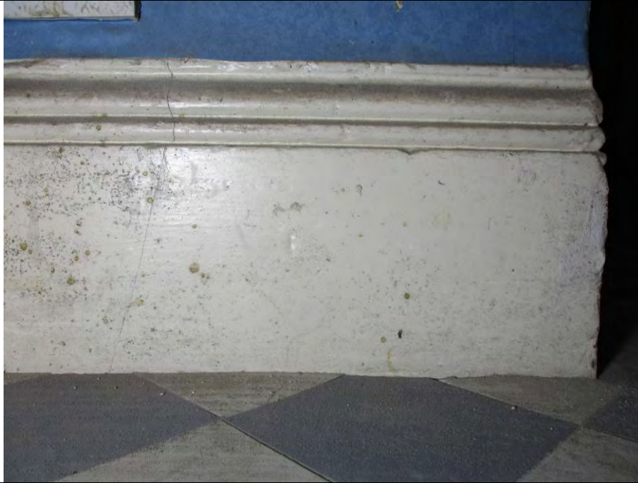
Room G1, showing profiled skirting.
