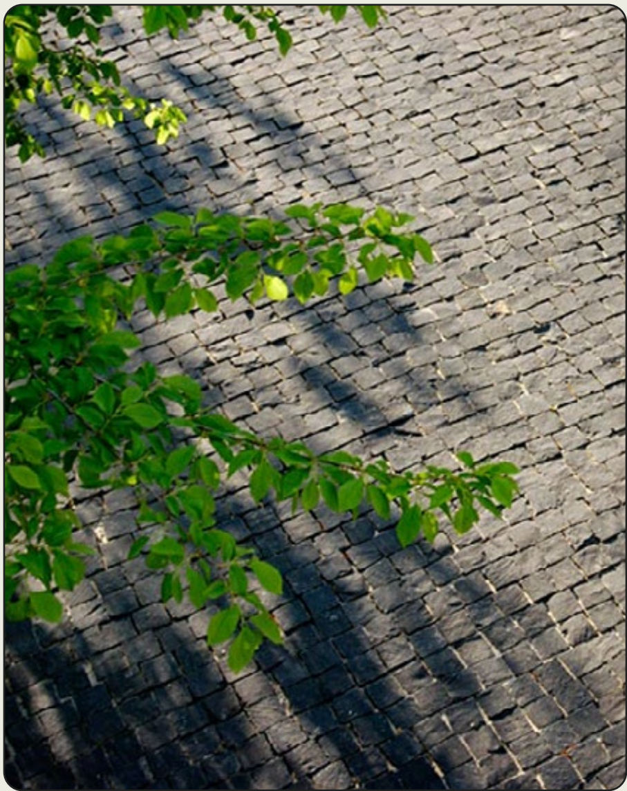
Setts laid with permeable bedding and jointing
