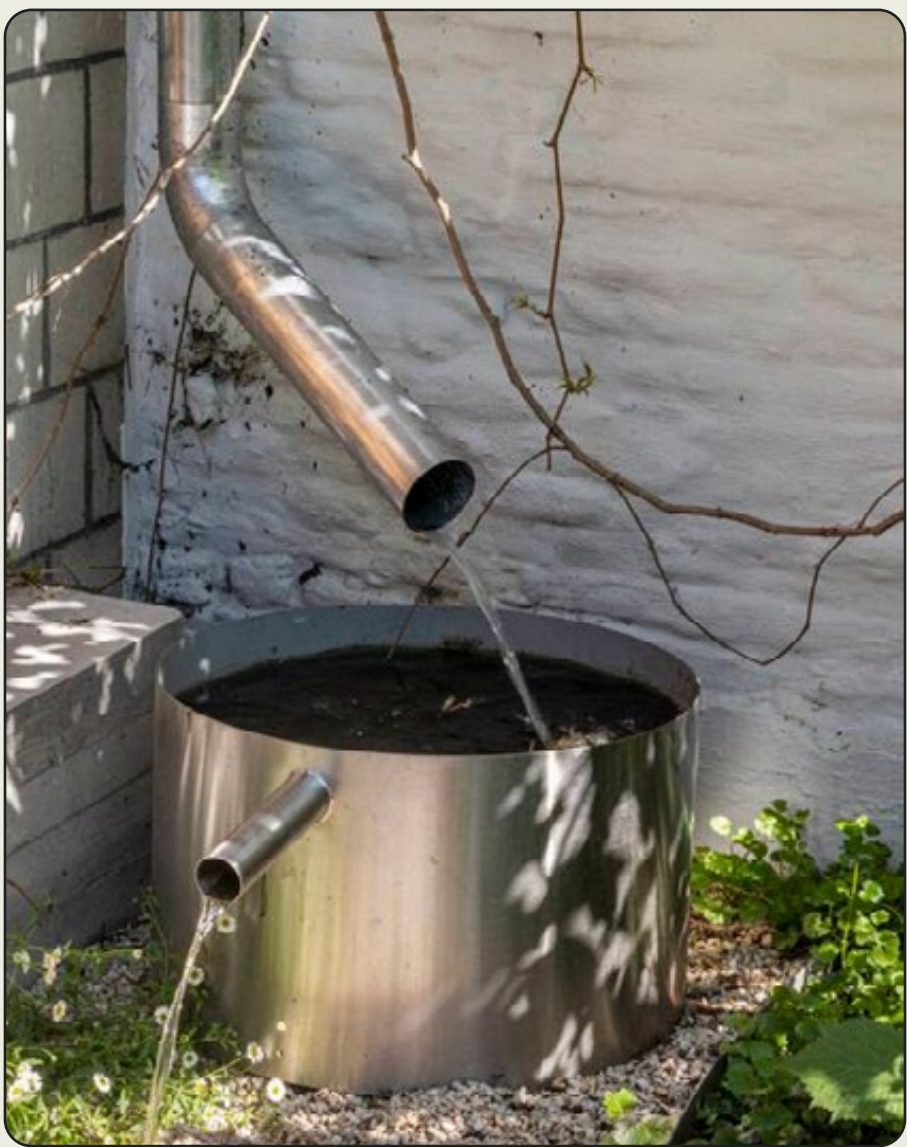
Bespoke rainwater SUDS planters
