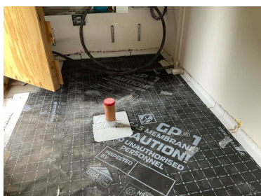
Overview of the infill installation to electrical room.
