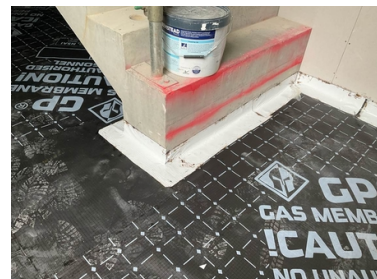
Retrofit termination detailing to stair core base using Juta GPSAM.
