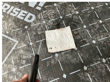
Probe testing to installers own CQA patch repair using Juta GPSAM.
