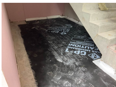
Overview of the infill installation to stair core area.
