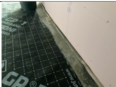
Overview of the infill gas barrier
