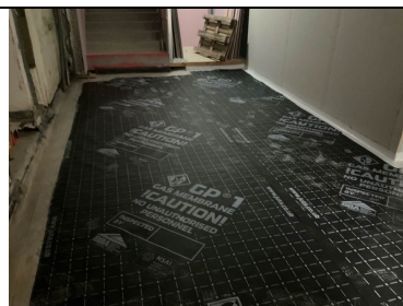
Overview of the infill installation to core area.
