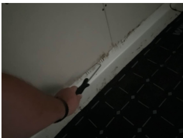
Probe testing to retrofit termination detailing along internal wall partition walls.
