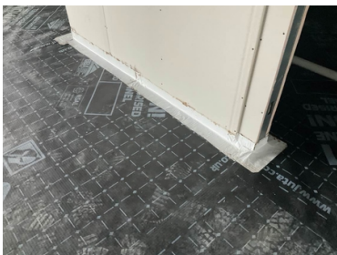
Overview of the retrofit termination detailing to internal wall partition walls.
