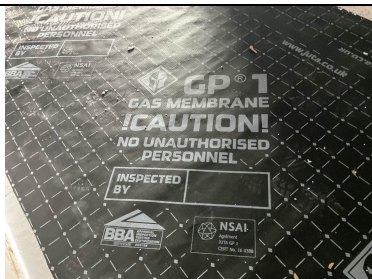
Evidence of Juta GP1 Gas Barrier installed on the project.
