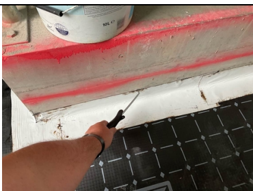
Probe testing along retrofit termination detailing to stair core base.
